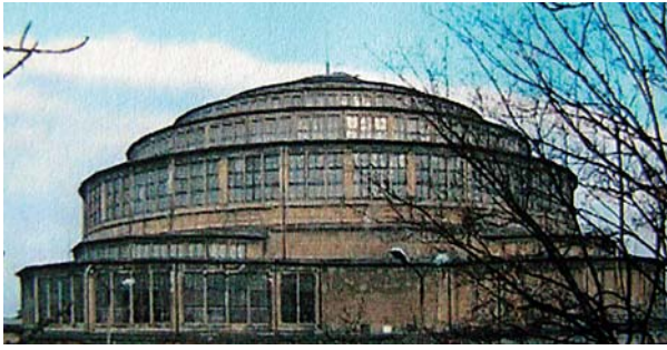
Ryc. 1. Widok Hali Stulecia we Wrocławiu przed remontem Fig. 1. View of the Centennial Hall in Wrocław before renovation
