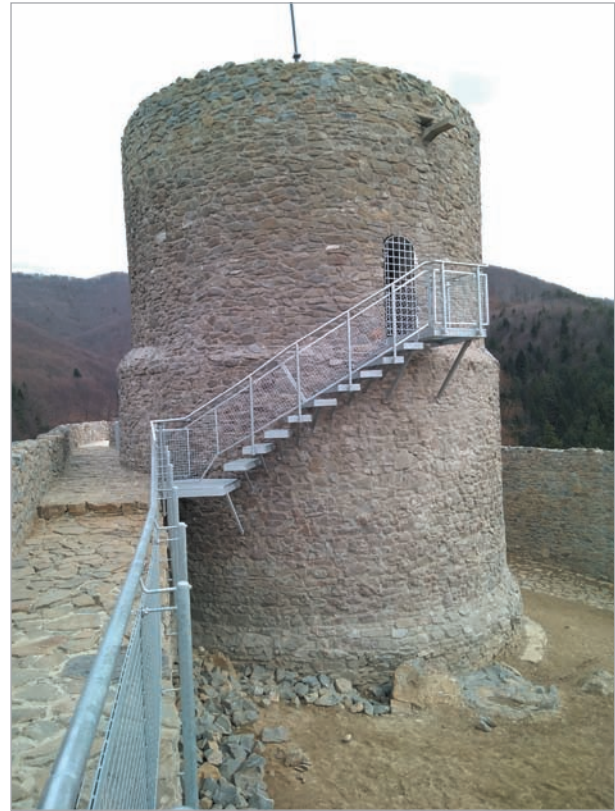
Fig. 14. The cylindrical tower in Rytro Castle, built at the end of the 13 th century; most likely a similar tower to the one that used function in Biecz (photo taken by P. Kocanda, 2018).
