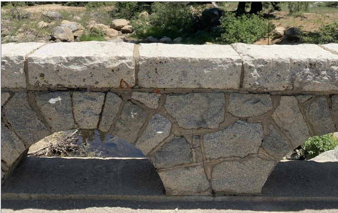
Source: Photograph taken by Ascent Environmental in 2021. Stone Railing of SR 89 Bridge over Meeks Creek
