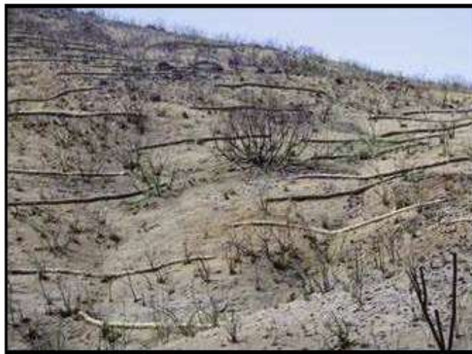
Figure 2B—Fiber roll placed across the hillslope. Not all the fiber rolls are on the contour which can accelerate erosion.
