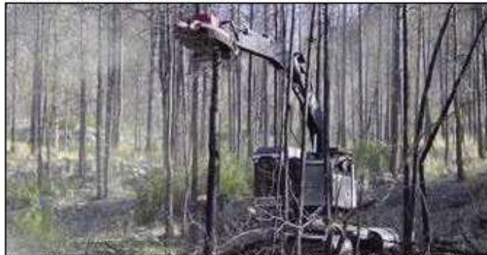
Figure 15—Mechanized equipment can quickly produce slash for effective soil cover.
