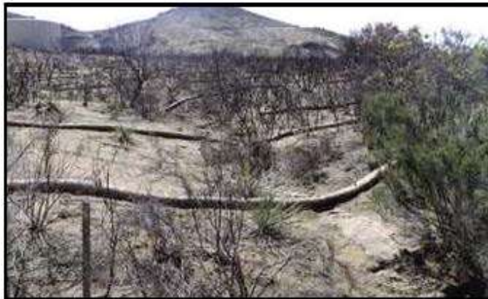
Figure 29—Avoid placing the fiber rolls in drainages.
