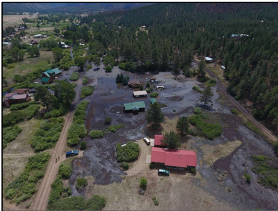
Figure 3.16. Aerial view of Ute Park area showing a post-flood debris flow after 0.3 inch of rain on July 13, 2018.
