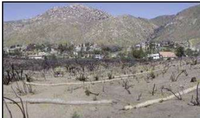
Figure 20—Fiber rolls do not reduce erosion but trap sediment on the slope. Where high values are at risk identify the emergency objective and select the treatment which best meets that objective.
