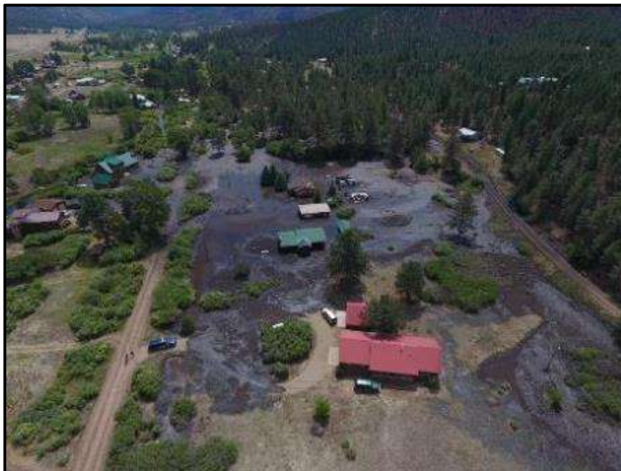
Figure 3.64. Ute Park post flooding, June 13, 2018, showing debris flow crossing two roads within the community.
