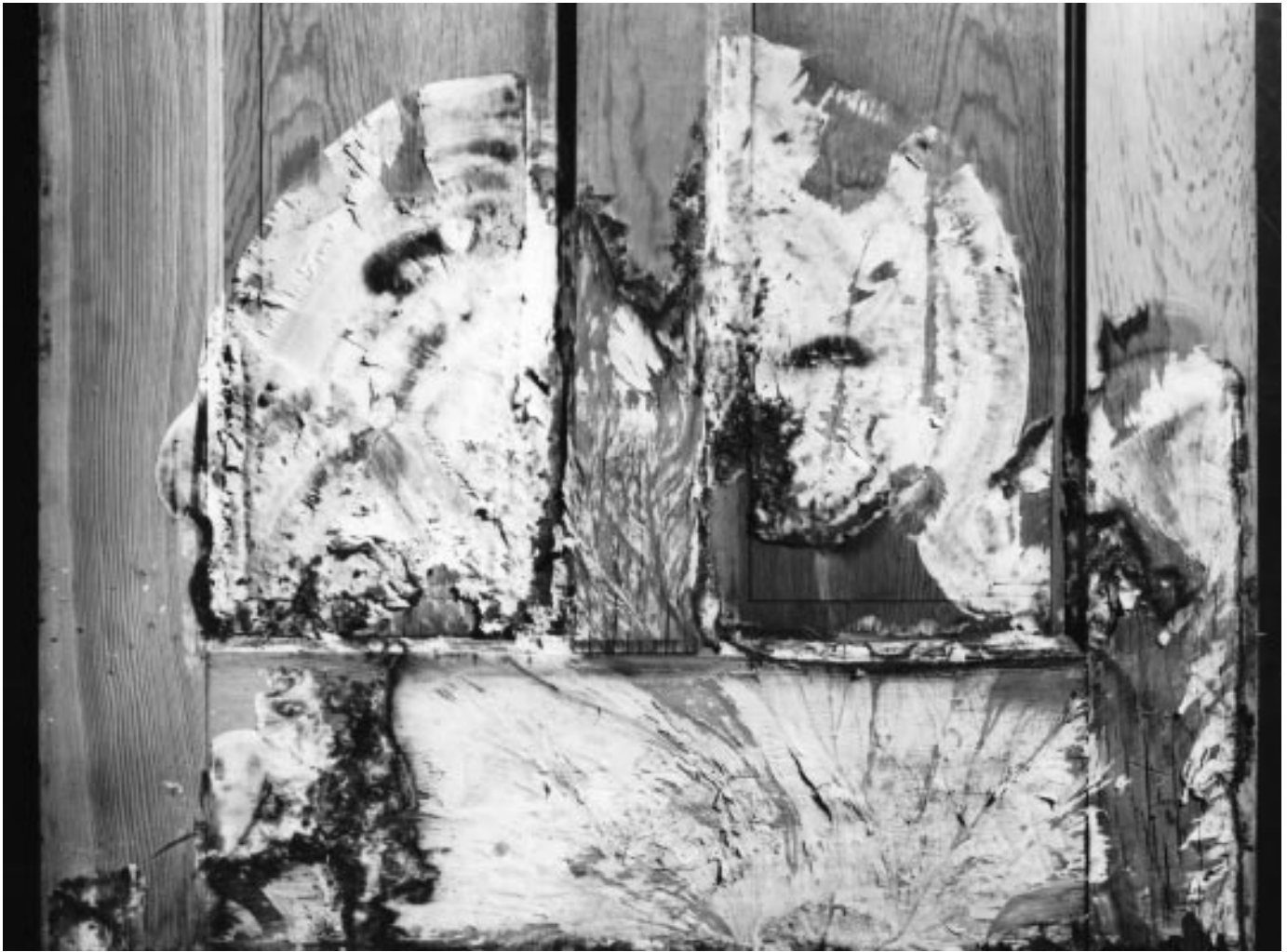
Figure 13–4. Mycelial fans on a wood door.
