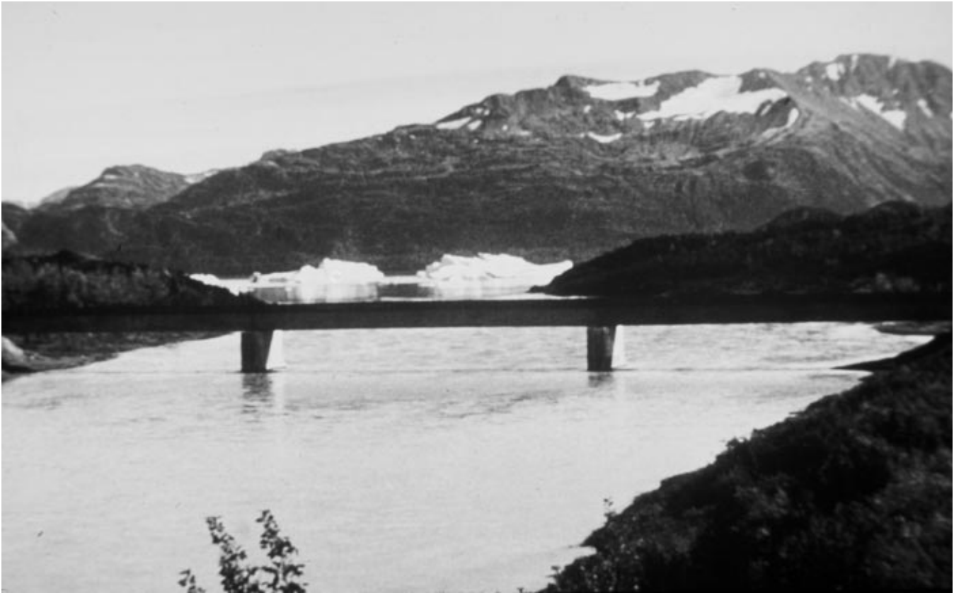
Figure 16–9. Glulam beam bridge over the Dangerous River, near Yukatat, Alaska, consists of three 43.5-m (143-ft) spans. Each span is supported by four 2.3-m- (91.5-in.-) deep glulam beams.
