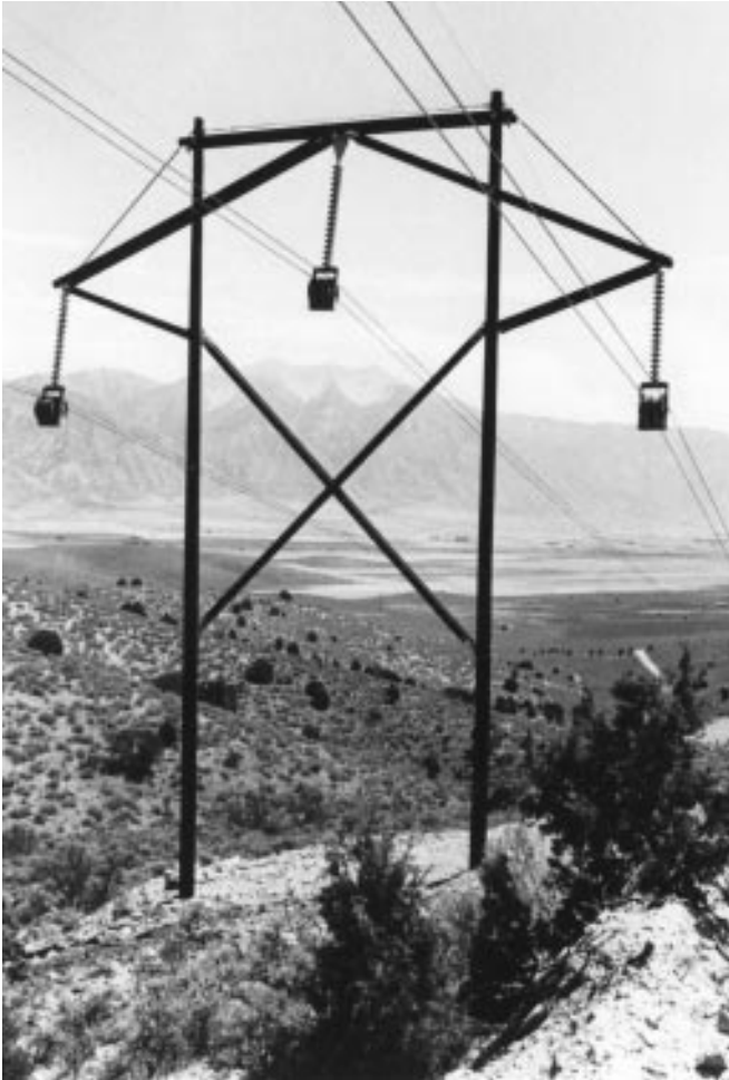
Figure 18–1. Round timber poles form the major structural element in these transmission structures. (Photo courtesy of Koppers Co.)
