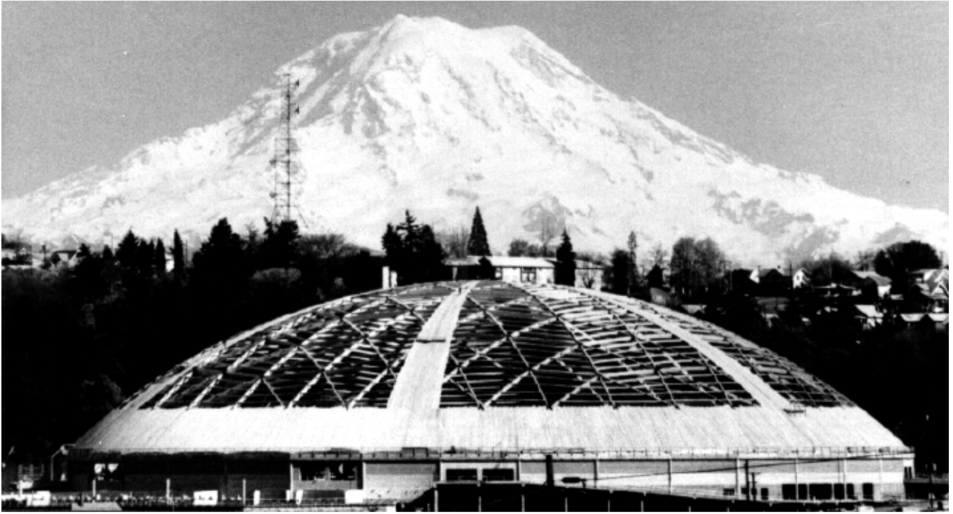
Figure 16–8. This 161.5-m- (530-ft-) diameter Tacoma dome (Tacoma, Washington), built in 1982–1983, is one of the longest clear roof spans in the world. (Photo courtesy of Western Wood Structures, Inc., Tualatin, Oregon.)
