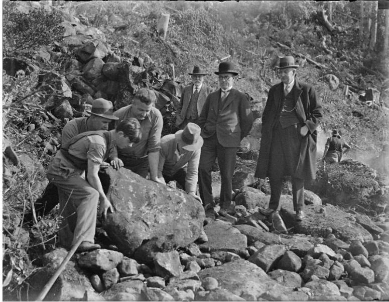
Above: Building Pinnacle Road, Mt. Wellington, with Premier A. G. Ogilvie and Mayor J. J. Wignall (AOT NS4023/1/51)
