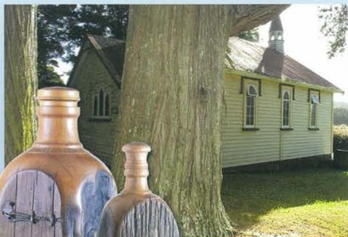
Below: Joinery in early buildings was most often made of heart totara. Chemical extractives in totara retard drying of normal primer paints and so special totara primers with low oil content were used.
