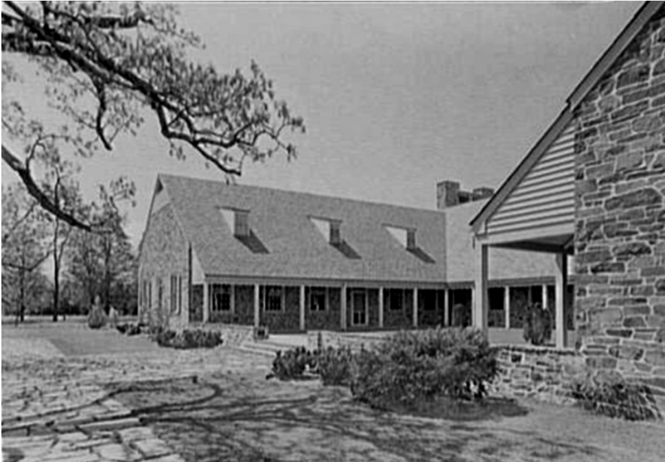
Figure 49: Historic view of the Library entrance plantings and courtyard lawn looking southwest, 1941. Also note flagstone walk and simple treatment of courtyard. (Digital image 5a07078r, Historic American Building Survey, Library of Congress American Memory Collection.)
