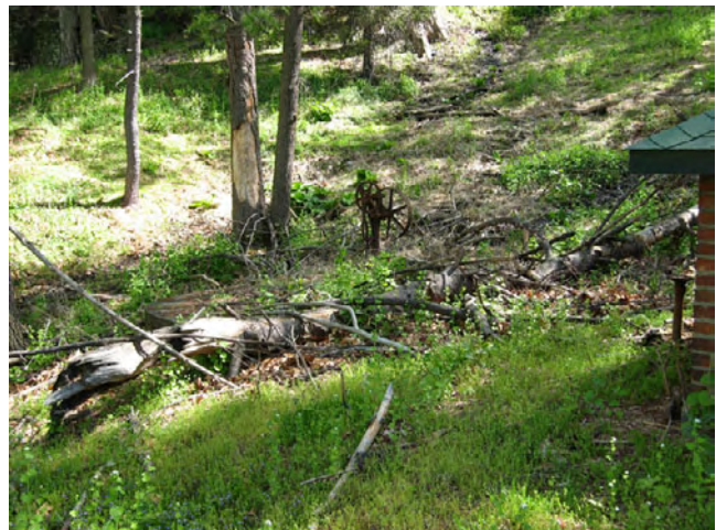
Figure 46 (right): Current view looking northeast uphill at the old reservoir showing its rusted gears and debris-strewn condition. At right is the corner of the pump house. (SUNY ESF, 2007.)
