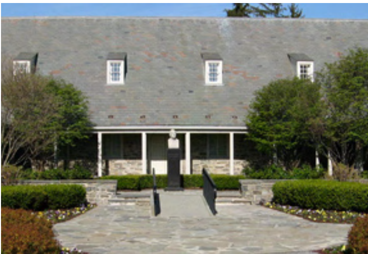
Figure 51: Recent view into the Library courtyard showing plantings made after 1971. (SUNY ESF, 2007.)
