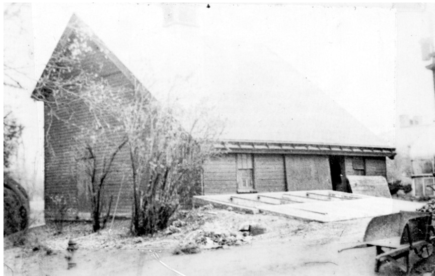
Figure 27: Photograph of the Large Ice House hotbed looking north taken soon after the end of the historic period in c.1946. Note the glazed sash in an open position. (Negative R-147, Roosevelt-Vanderbilt National Historic Sites.)
