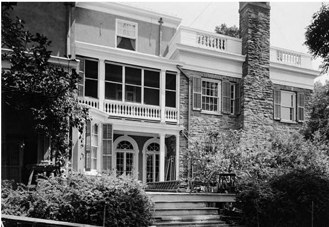
Figure 21: Historic view looking east at the plantings along the west deck, July 1941. To the left of the steps is a clipped spirea hedge; to the right is a mass of barberry and spirea. Honeysuckle is growing on the west porch column at left. (Digital image 115850pr, Historic American Building Survey, Library of Congress American Memory Collection.)
