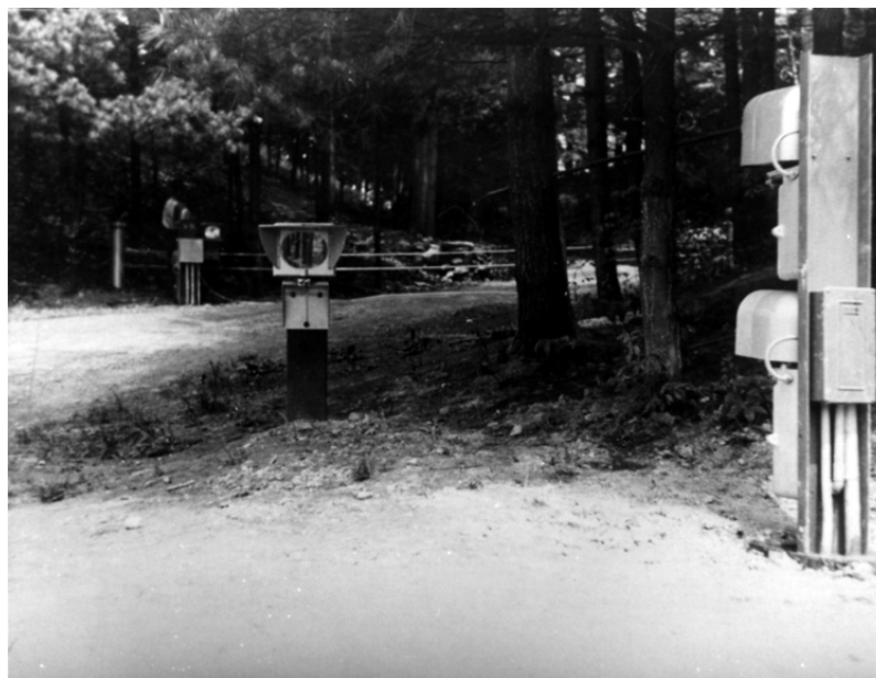
Figure 39: Historic view looking northeast from the intersection of River Road and the Duplex Road showing war-time security system (electronic eye, crash barrier), c.1942. Remnants of this system remain at this location. (Photograph px 80-26:44 (8), Roosevelt-Vanderbilt National Historic Sites.)
