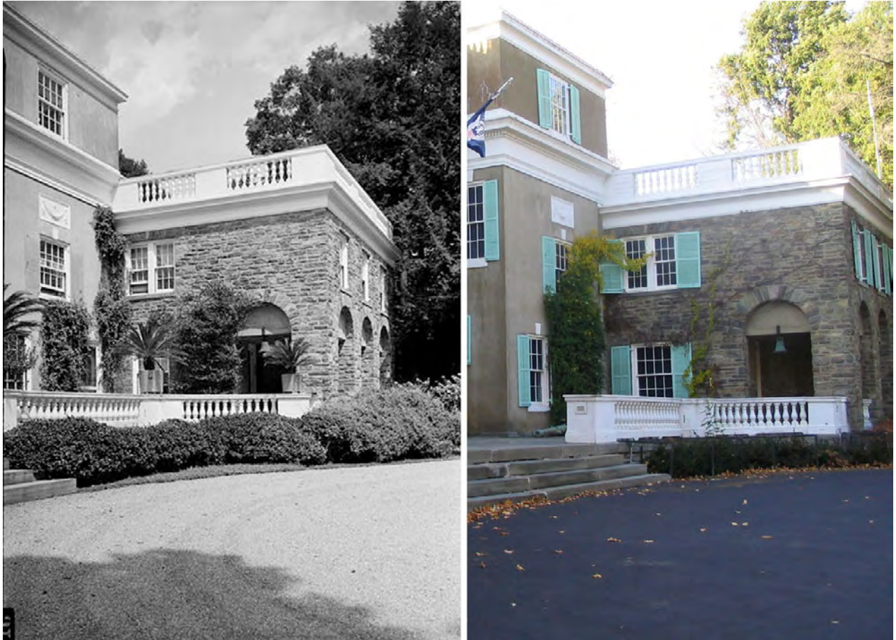
Figure 8: Comparison of paving character showing gravel-surfaced turn-around in July 1941 and the existing black asphalt that replaced it. These images also changes to the foundation shrubs. (Left: Digital image 115847pr, Historic American Building Survey, Library of Congress American Memory Collection; right: SUNY ESF, 2005.)
