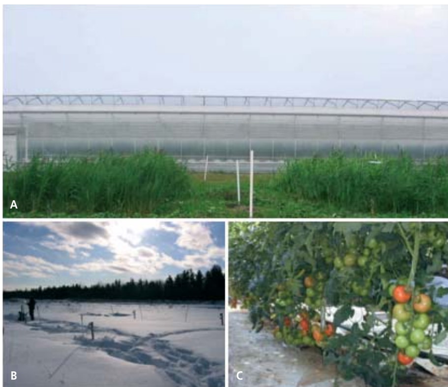
Figure 2. A) Vertical subsurface flow constructed wetlands built at a commercial greenhouse facility (Les Serres Nouvelles Cultures - Sagami, Ste-Sophie, Quebec, Canada) to treat tomato effluents; B) A lower distribution level located at a depth of 0.6 m is used during the winter time, and the top one during the summer season. A meteo station collects air and soil temperatures at different levels of the constructed wetlands (CW) as well as the rain water; C) A tomato crop grown into an organic growing medium where the effluents are collected and treated via the CW.
