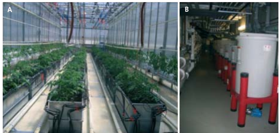
Figure 3. A) Organic growing system at Laval University (Quebec city, Canada) where effluents of 6 types of soil (replicated 6 times, total of 36 units) are independently monitored and recycled to the crop; B) Collecting reservoirs located at the basement of the greenhouse where effluents are individually monitored and pumped back to the crop to eliminate nutrient and water emissions into the environment.
