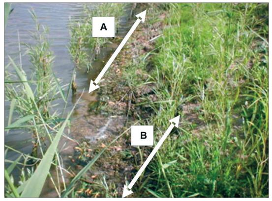
Fig. 7: The condition of the bank after 5 months – the bank retreat of the comparative area is apparent with vigorous growth of willows and a very good effect of the proposed stabilization: A) stabilized by geonet, B) without geonet – the Bílovec reservoir, Moravia, Czech Republic (photo: M. Šlezingr)
