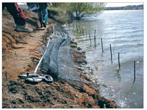
Fig. 6: Geonet was attached to the bottom range of Salix fluviatilis rods 0.7 m in length. Subsequently, geonet stabilized the slope of the same kind of willow cuttings in four rows. In conclusion, we stabilized the slope by a layer of soil of about 3 cm and sown grass mixtures (photo: M. Šlezingr)
