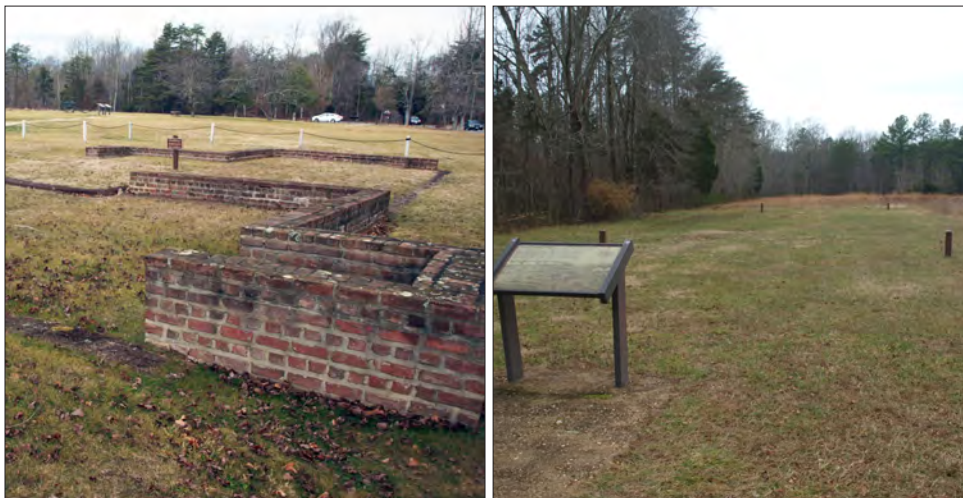
Figure 3.16. Examples of contemporary brick foundation footprints and building corner posts that could be used to interpret the site of the Val-Kill tenant farmhouse. These examples are from Fredericksburg & Spotsylvania National Military Park in Virginia. (SUNY ESF)
