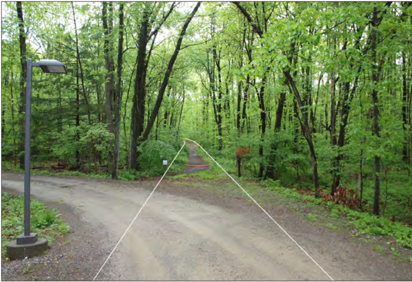
Figure 3.18. The road to Top Cottage looking east from the historic core showing erosion of roadbed into a narrow trail, 2012. The white lines indicate the limits of the recommended reestablished roadbed, including the section enlarged by current vehicular use. (SUNY ESF)
