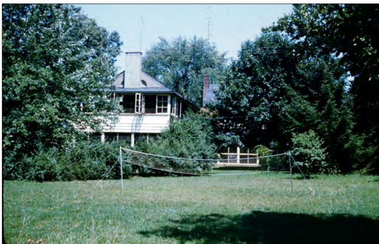
Figure 0.4. Mrs. Roosevelt's cottage, showing wing added to the original factory building (section in right background), looking east, ca. 1945. (Dickerman Collection Slides, Roosevelt-Vanderbilt National Historic Sites)
