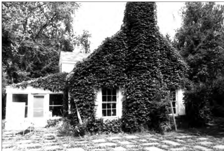
Figure 0.6. Stone Cottage and the pool terrace patio showing years of neglect prior to restoration, looking north, 1978. (Roosevelt-Vanderbilt National Historic Sites)
