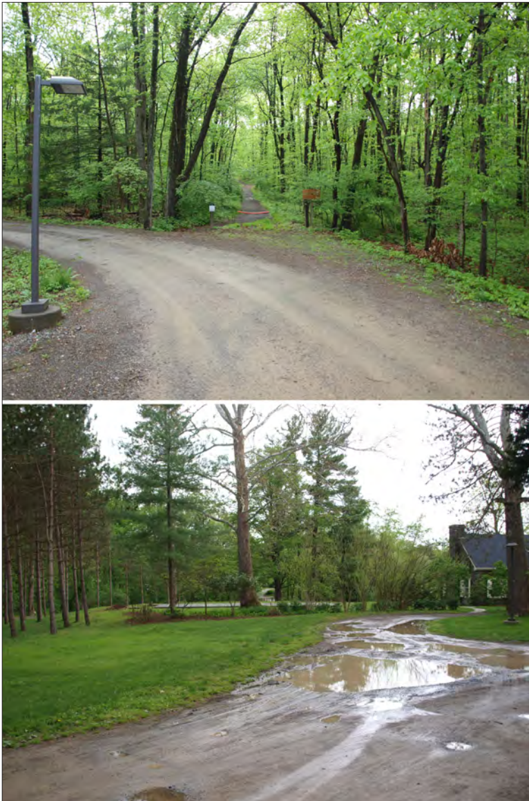
Figure 2.5: Deteriorated condition of Val-Kill roads, showing the road to Top Cottage (Hyde Park Trail) looking east with its segmented and narrowed roadbed (top), and the loop drive at Stone Cottage, looking west with its eroded surface and edges, 2012. (SUNY ESF)
