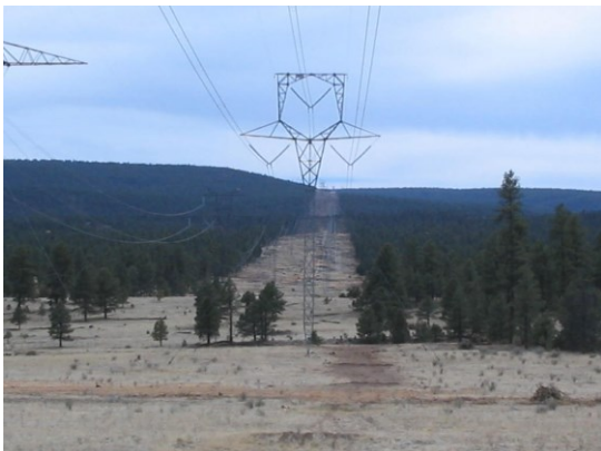
Cleared transmission right of way near Luna, NM. © Nick Smokovich/NMFD
