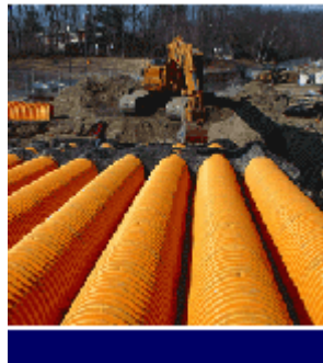
Stormtech Chambers being installed (Stormtech 2004)
