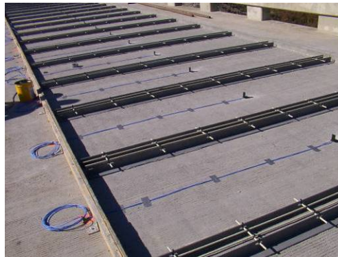
Electrode Arrangement (Tuan 2004a)
