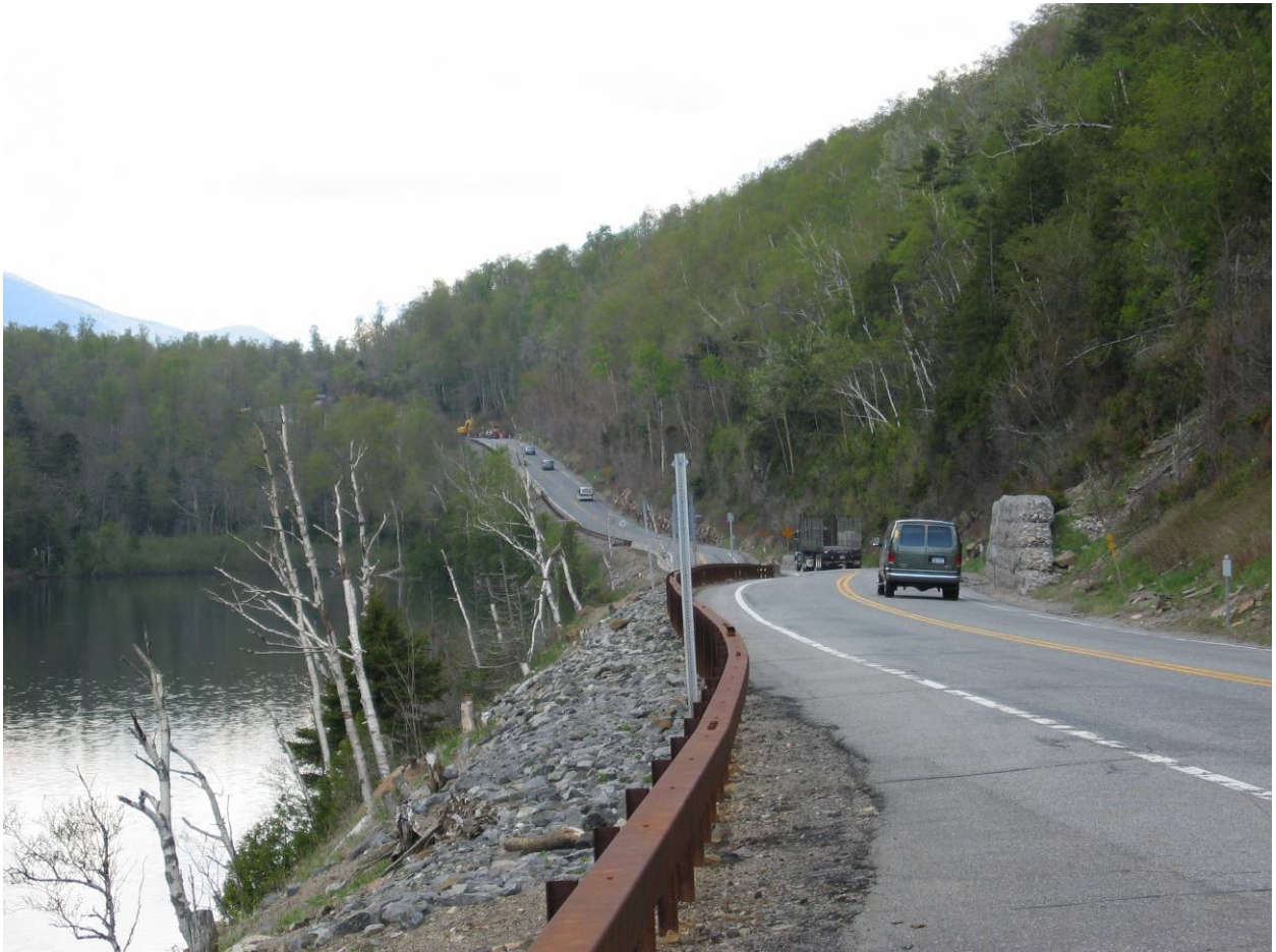
Route 73 at Upper Cascade Lake, looking west. Photo by Kerop Janoyan.
