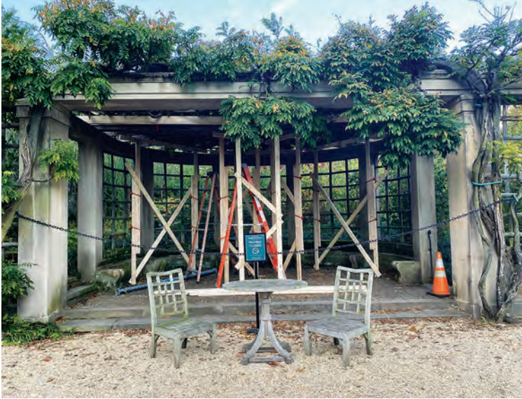
Pebble Garden Arbor braced for construction.
