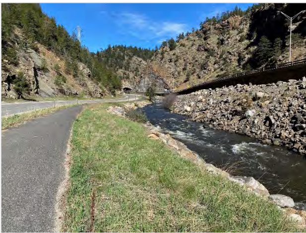
Photo 23. Looking west along the East Idaho Springs Road/I-70 Frontage Road, south of I-70 and east of the Veterans Memorial Tunnels near MP 242.6 in May 2020. Example of sparsely vegetated slopes north of I-70 and more forested slopes south of I-70 and Clear Creek. Narrow vegetated buffers exist between the frontage road and the Clear Creek Greenway and Clear Creek.
