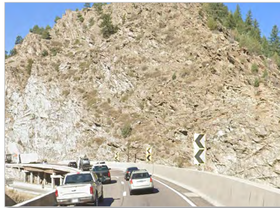
Photo 3. Location of Westbound Entrance of Proposed Tunnel
