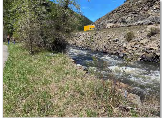
Photo 30. Picture looking west from the Clear Creek Greenway near MP 243.7 in May of 2020. Example of sparsely vegetated slopes and narrow riparian corridor south of I-70. The several straight sections of Clear Creek in the "W" section of the highway provide rapids preferred by local white-water rafting companies.
