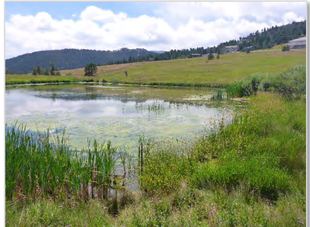
Photo 8. Looking south from the I-70 highway right of way, east of the Hyland Hills/Floyd Hill interchange. A large water quality pond is shown that drains into Beaver Brook to the east near MP 247 during the Summer of 2017.
