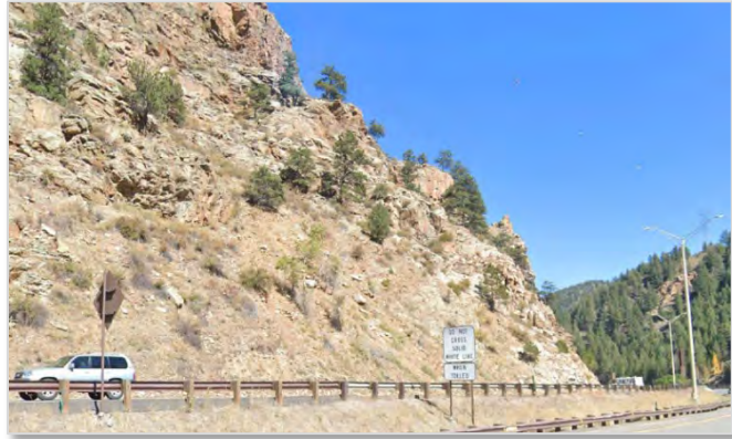
Photo13. Rock Cut Area, North Side of I-70
