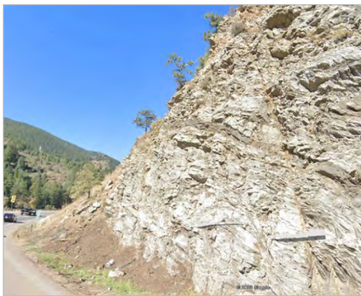
Photo 4. Rock Cut Area, MP 244, Looking West
