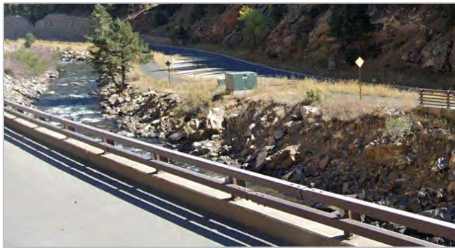
Photo 15. Clear Creek Realignment Area
