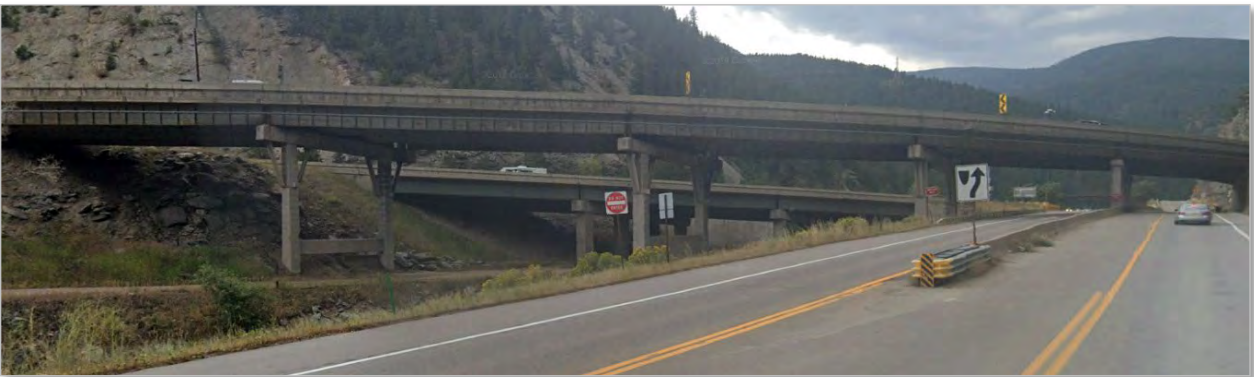
Photo 1. I-70 Westbound Bridge—Bottom of Floyd Hill
