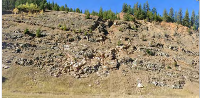
Photo 2. 200-Foot Tall Rock Outcrop, South Side of I-70
