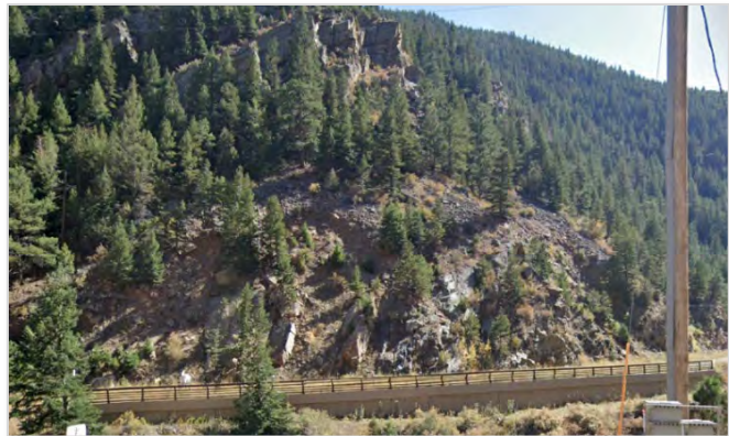
Photo 14. Rock Cut Area, South Side of I-70
