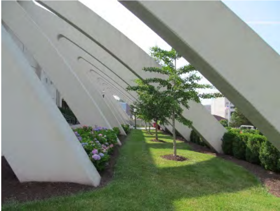
Figure 4-6 Support arches at Virginia Tech Stadium. (Courtesy Carol King)
