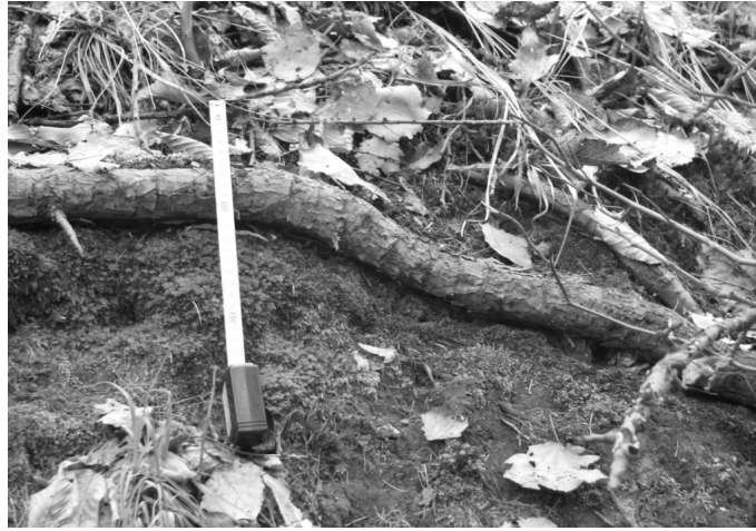
Figure 5: Example of exposed root on the slope of Samborowiczki gully system.
