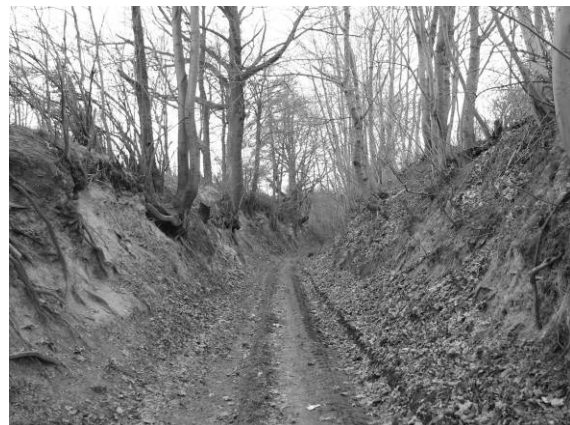
Figure 2: Erosion on the slope of the road gully, SW Poland
