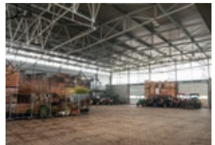
Works inside the hall can be performed throughout the year.
