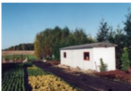
White house – the first rest and refreshment facility (lunchroom) at the Nursery by the main communication route, present up to date. Around 1996
