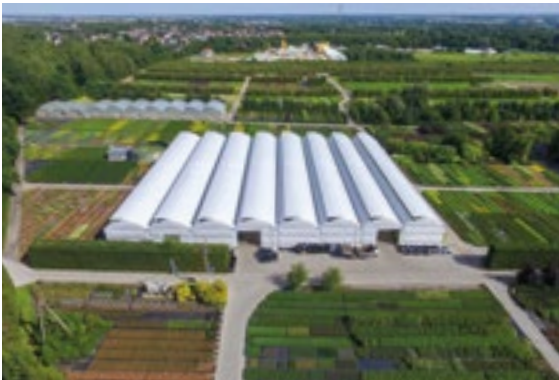
New tunnel block. 2019
