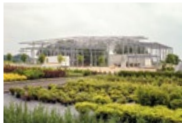
Production hall in the course of construction. 2003
