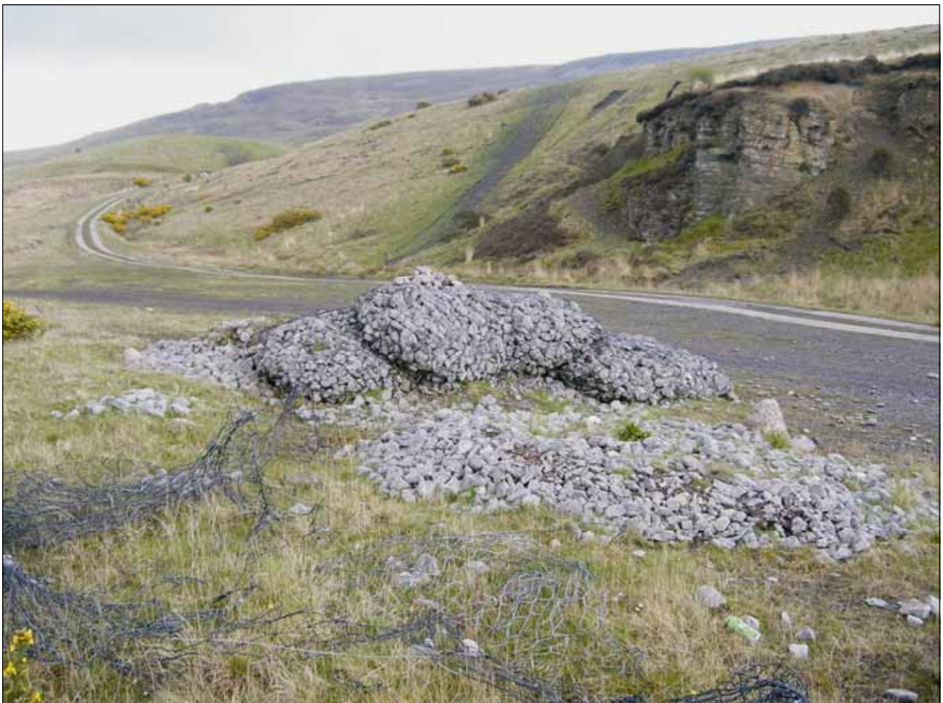
Mynydd Bach with discarded gabion. Photograph © Simon Warmingham
