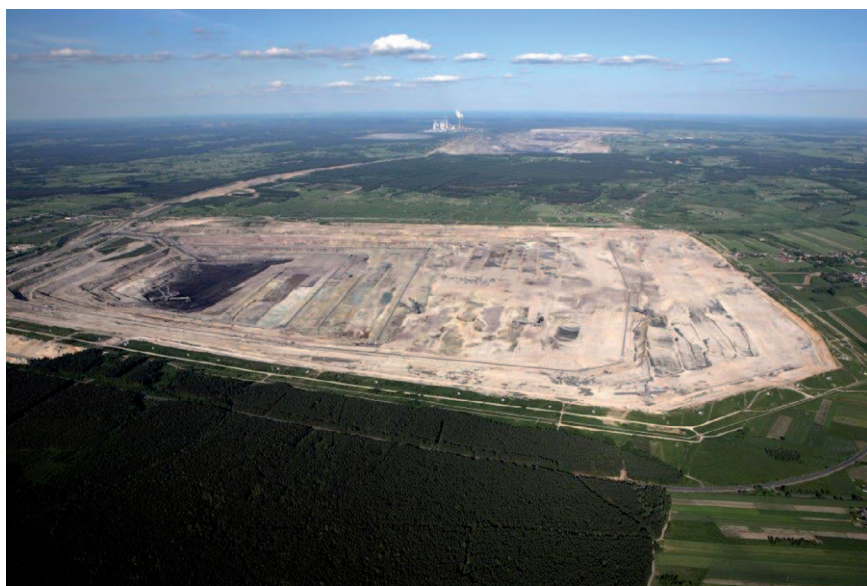
Photo 3.3. ‘Szczerców’ Field open pit – Archive of the KWB Bełchatów
