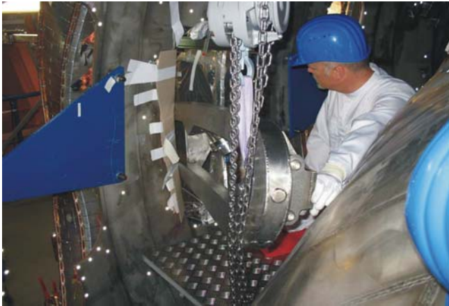
Figure 23: Assembly trials with in-vessel components (sweep coils)
