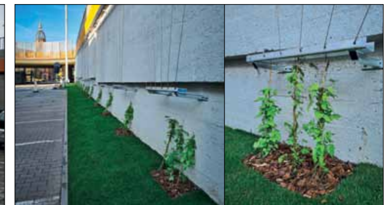
Figure 11.8 Green roadside in Chorzow — after. Photo: A.Beryt
