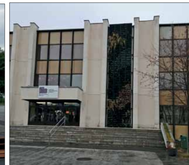
Figure 11.2 Green wall in Liptovský Mikuláš — after. Photo: P. Starek
