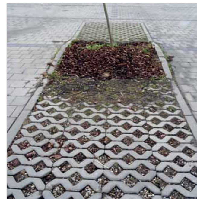
Figure 4.4 Tree planting as an element of UEA – green pavement. Photo: I. Tichá
