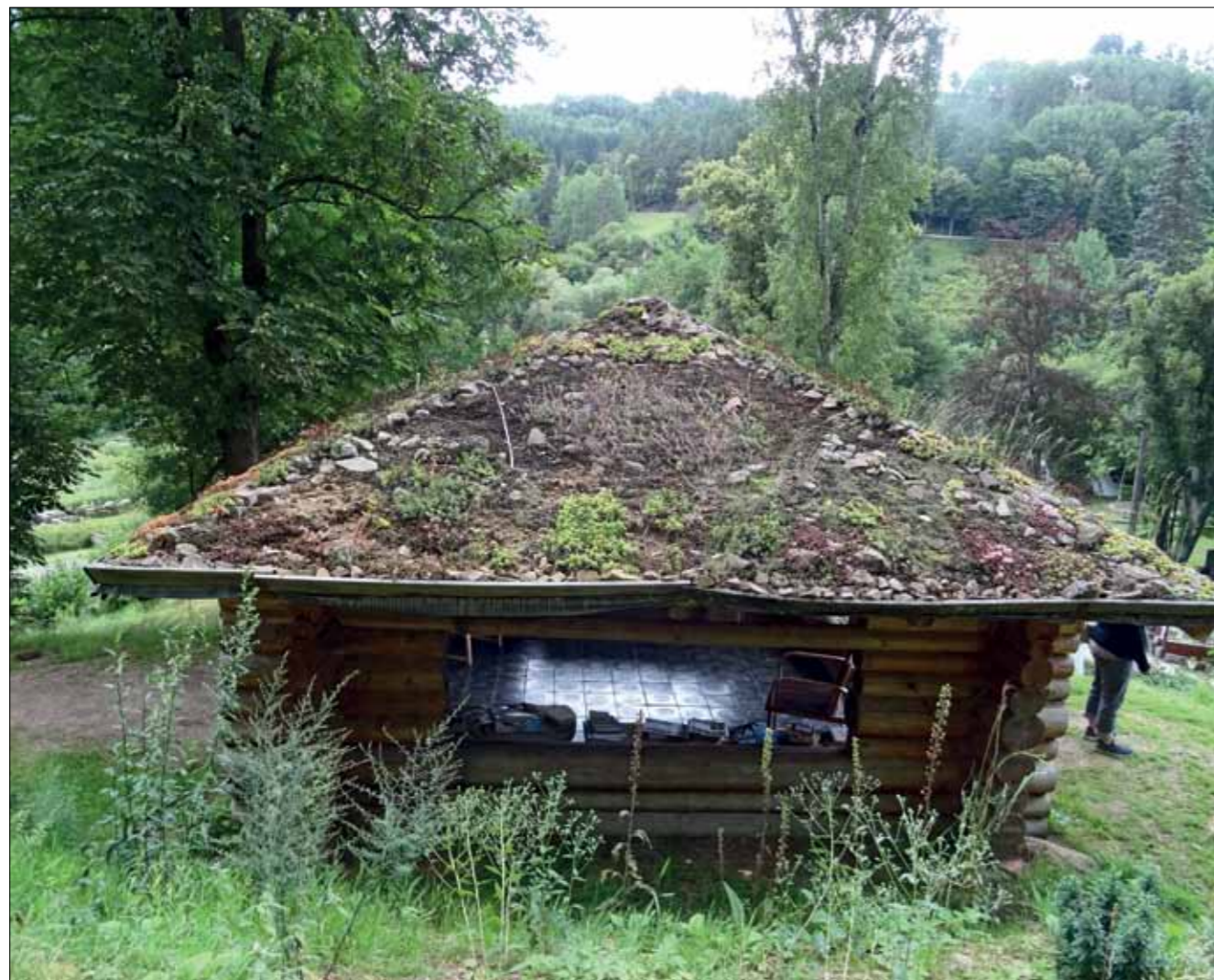
Figure 7.1.29.1 Green covering shelters. Photo: B. Vojvodíková
