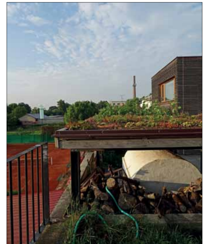
Figure 4.9 Green roof on a small shelter. Photo: B. Vojvodíková
