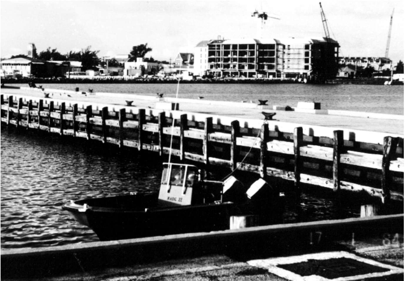
Figure 1–2. Wood is favored for waterfront structures, particularly fendering, because of its shock-absorbing qualities. The fendering on this dock in Key West, FL, is made of creosote-treated Douglas-fir ( Pseudotsuga menziesii ). Some tropical species are resistant to attack by decay fungi and marine borers and are used for marine construction without preservative treatment.
