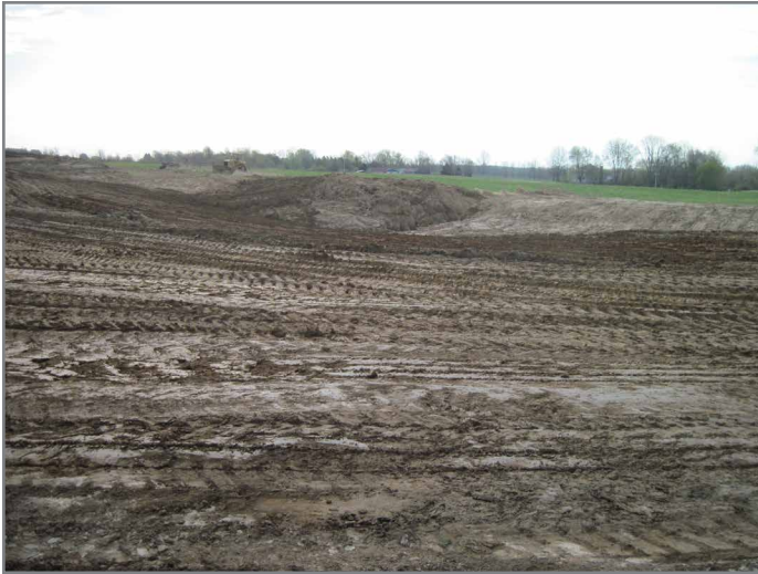
Drained farm pond being filled, Union County, Illinois (JG Palis).
