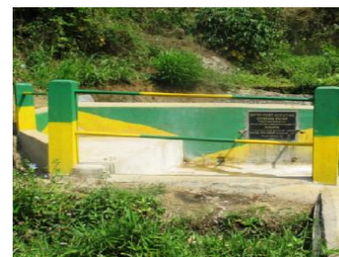
Figure 7.8: RCC Water Storage Tank for Drinking Water
