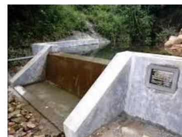
Figure 7.9: Spring Tapped Chamber
