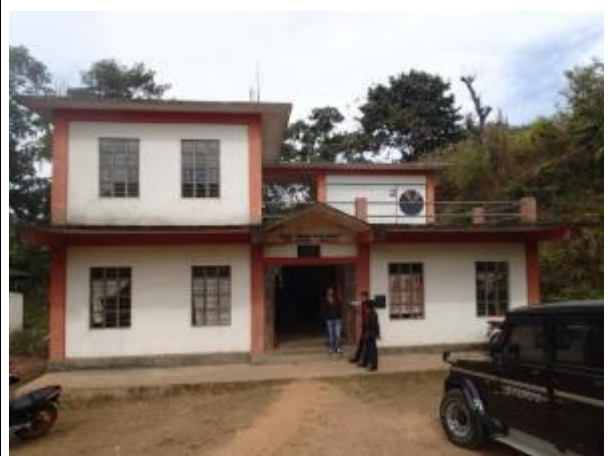
Exterior of Enterprise Facilitation Center building of Megha-LAMP in Mawshynrut CR&D Block, West Khasi Hills District
