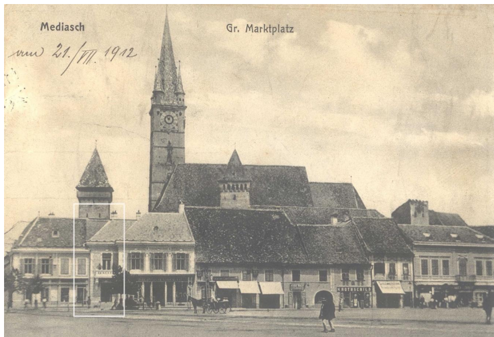
Fig. 7 11 . The facade and the roof are reshaped before 1912. The wall of the Trompeterthurm tower can be seen throughr the emptiness released by the new roof that apparently violates the building regulation.
