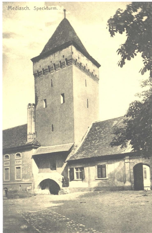
Fig.9 14 . Square front with gutter but without downpipes
