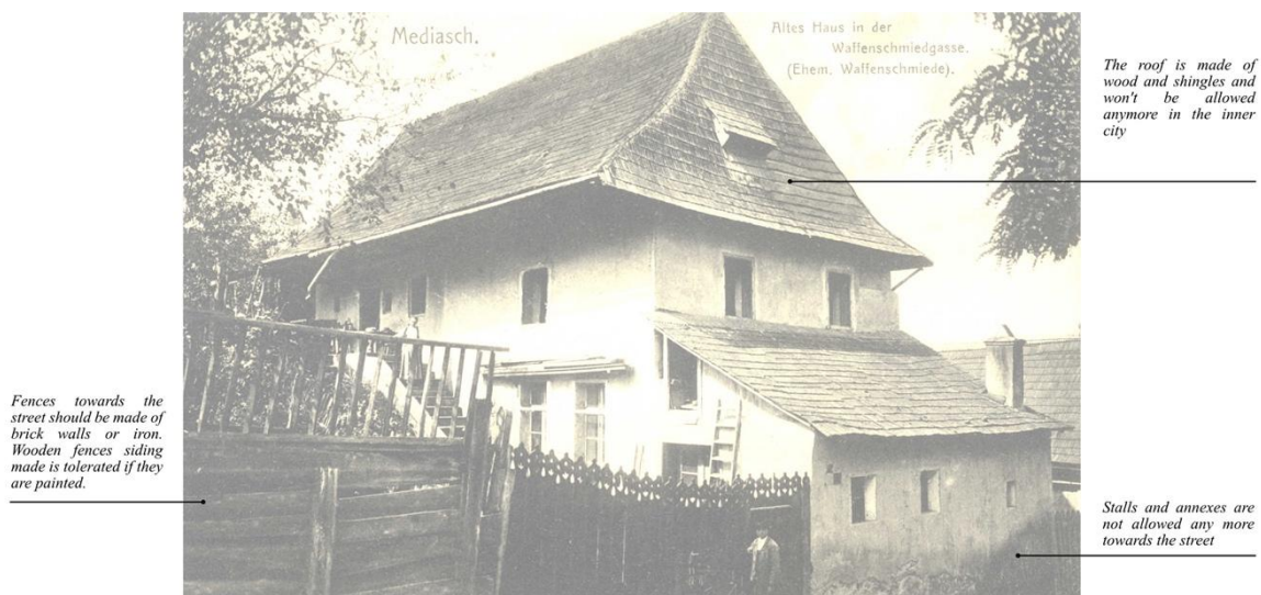
Fig. 11 16 . Old house of former gunsmith was probably impressive too for the generation that has taken the picture. The house reveals some elements that will be eliminated by the building regulation at the end of the 19th century.
