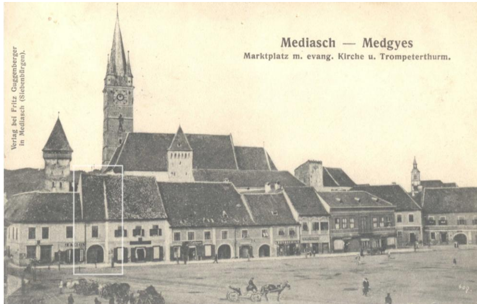
Fig. 6 10 . The central square. The roof shape of the second building before intervention is constructed with fire wall but paradoxical it will be shaped in a way that conducts rainwater towards the neighbour.
