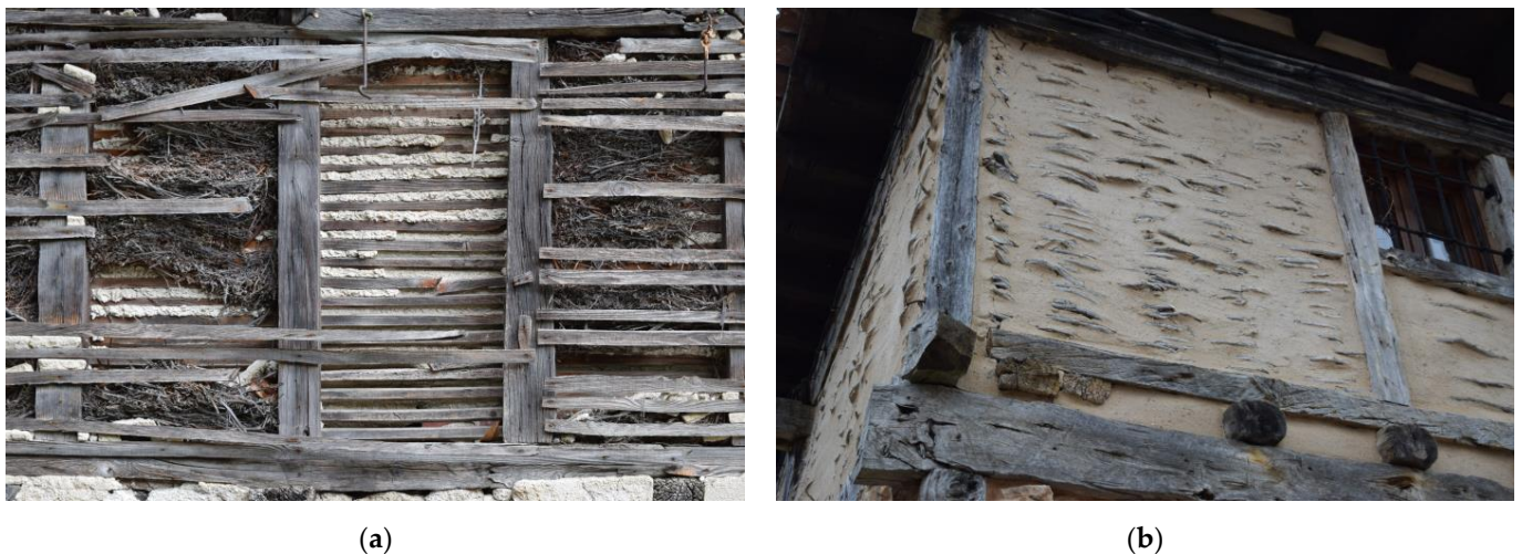
Figure 2. Examples of half-timber walls with lightweight screens: (a) rigid screens of lath-and-daub in As Ermidas (Ourense); (b) flexible screen of wattle-and-daub in Calatañazor (Soria).
