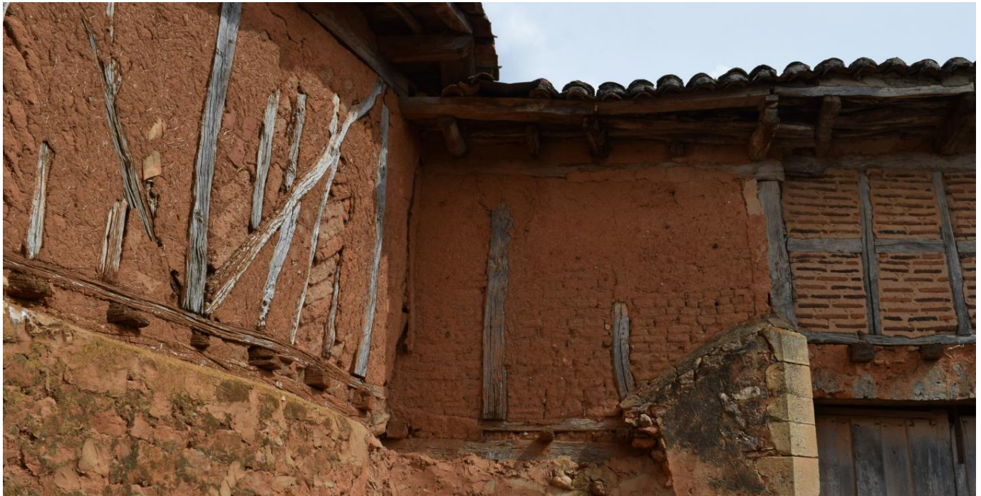
Figure 25. Half-timber wall with heavy adobe filling, where the wood used for the construction of the framework must meet minimum mechanical resistance requirements. Building located in Pedro de Ojeda (Palencia), with the sample PA1 analysed and identified as belonging to the Populus genus.
