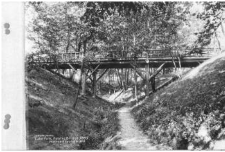
Original Rustic Bridge
