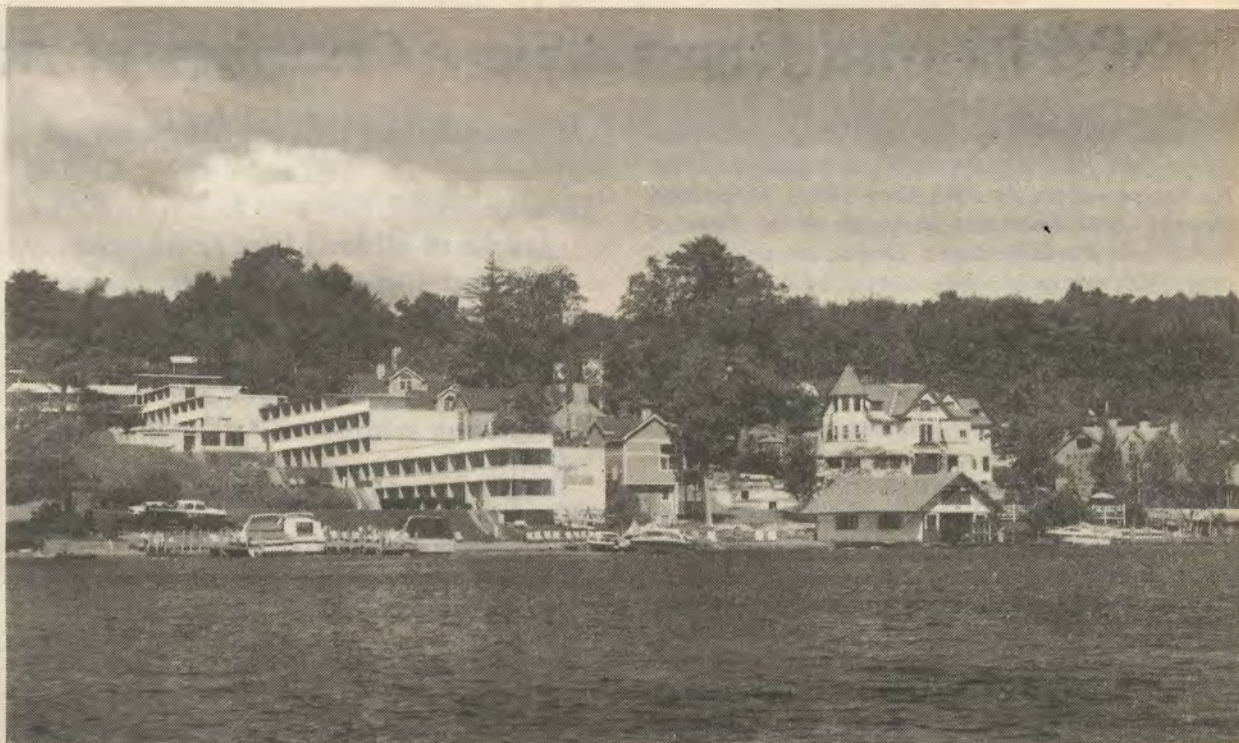
Shoreline development, such as Tahoe Resort on Lake George, threatens some of the most beautiful, undeveloped tracts in the Adirondack Park. Backcountry development of forestland, while less visible, is equally threatening. Local residents of the Park do not see the profits generated from this sort of development project. Can the APA protect the Park's ecological integrity? Photo © Alan Cederstrom, courtesy The Adirondack Council
