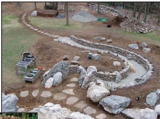
The construction begins.
