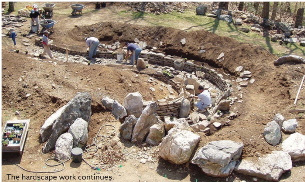
Workers lay out the hardscape.
