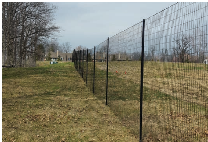
Armor-Flex fence used in the Cleveland, OH, Metro Parks.
