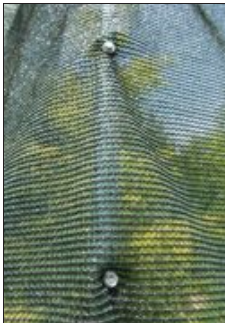
The screen with cable tie eyelets.
