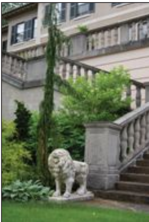
A close-up of the base of the grand terrace. Photo by Elmer Dustman
