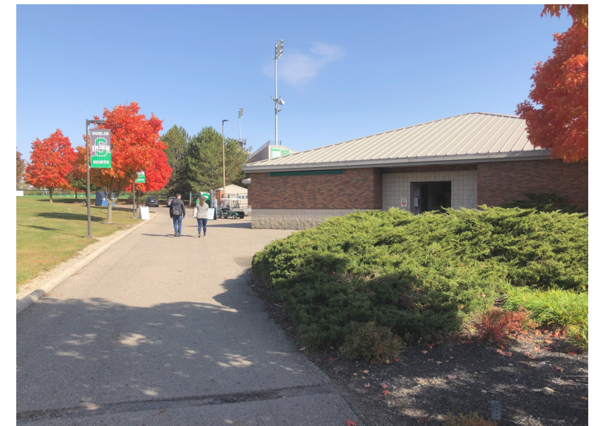
Existing View of Football Concessions West
