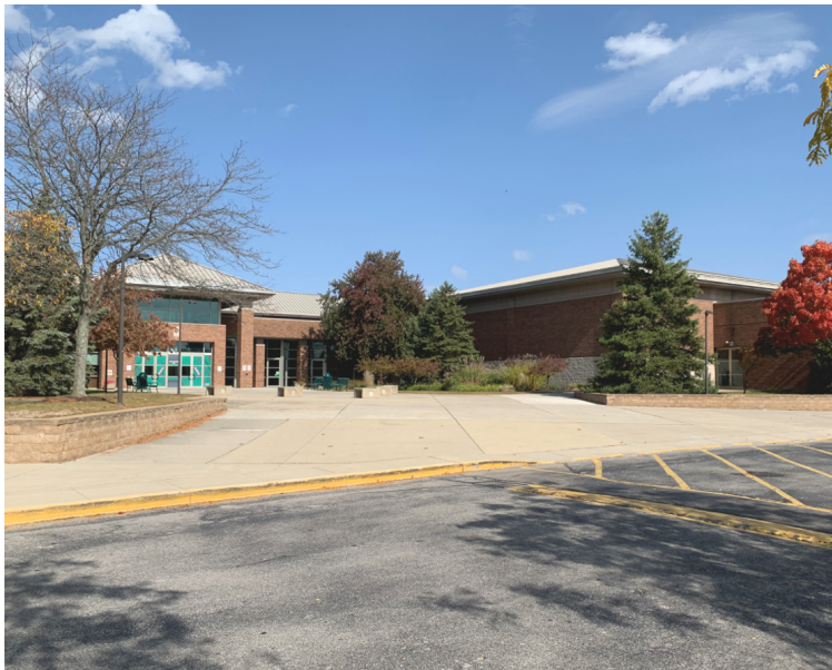
Existing Views of High School Building
