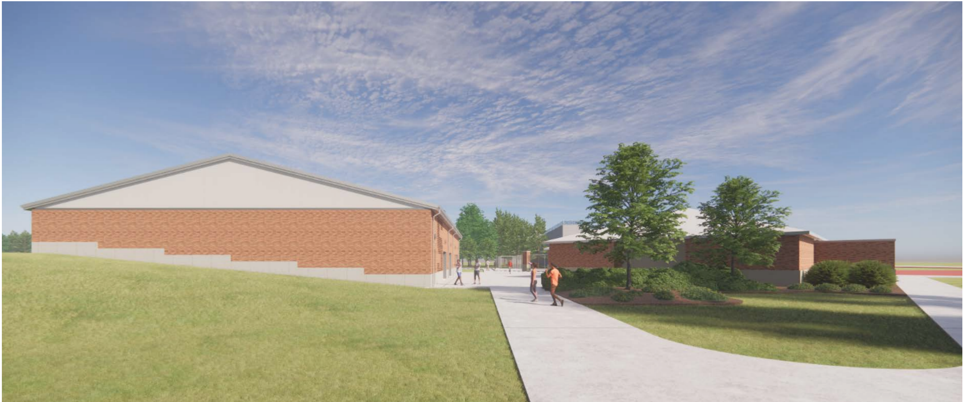
View Looking North at New Multi-Use Athletic Facility
