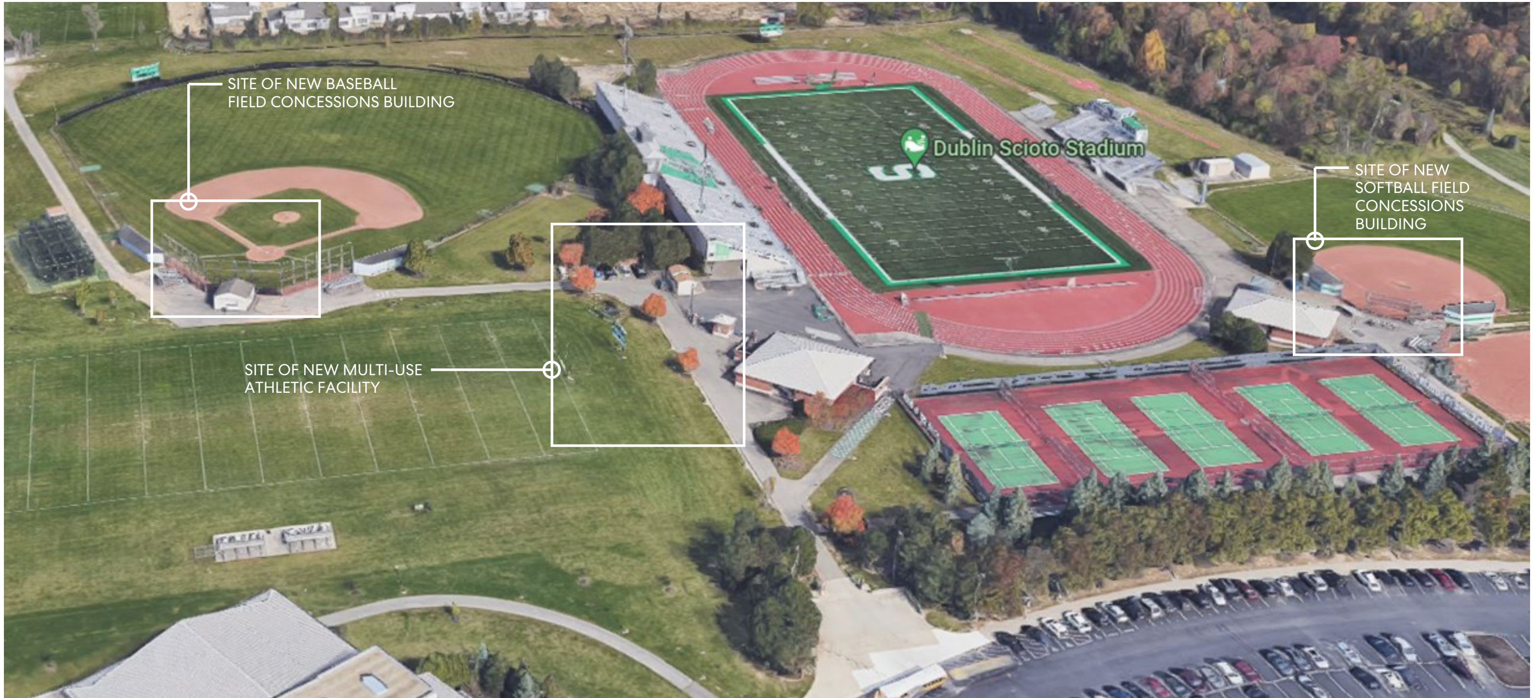
Aerial view of Existing Athletic Facilities
