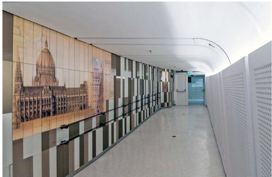
Final constructed tunnel
