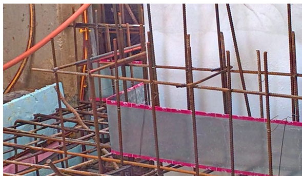
Cast in place walls being formed with typical joint waterstop detail to left
