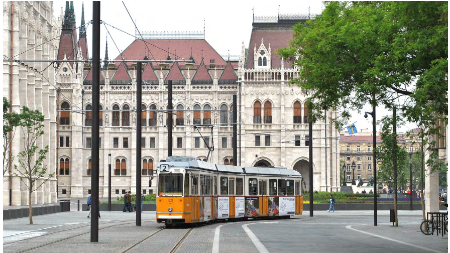
Street car line running over top of the tunnel
