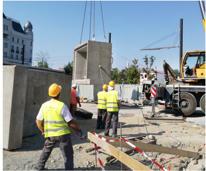
Precast sections and their installation
