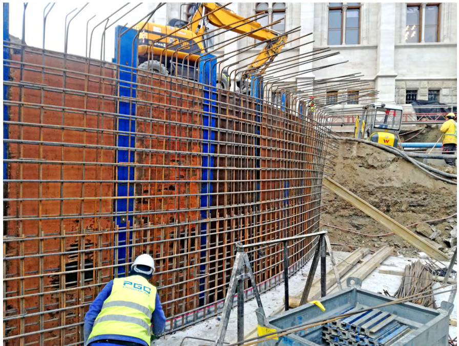
Cast in place walls being formed with typical joint waterstop detail to left
