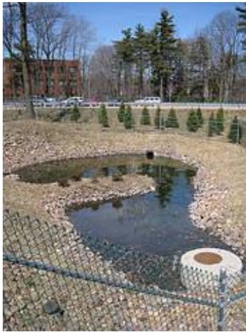
Hinesburg Rd. Stormwater Utility
