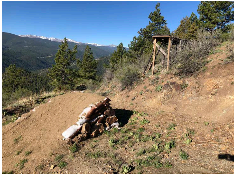
Existing Dilapidated Rogue Trail Features
