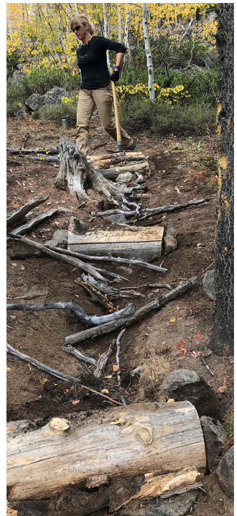
A Decommissioned Trail With Check Dams
