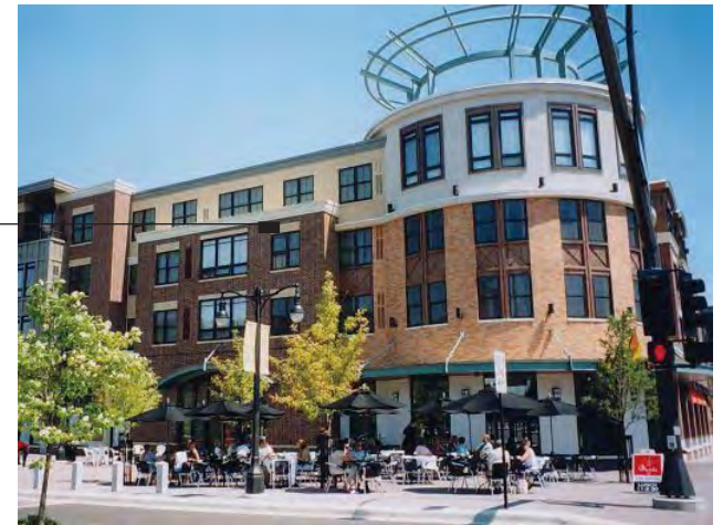
Mixed-use building with distinct top, middle, and ground floor, distinct horizontal modules, interesting corner treatment, a variety of window shapes and decorative awnings.
