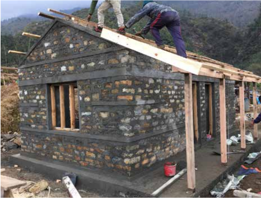
Locally employed civilians repairing the roof of a home © Crown
