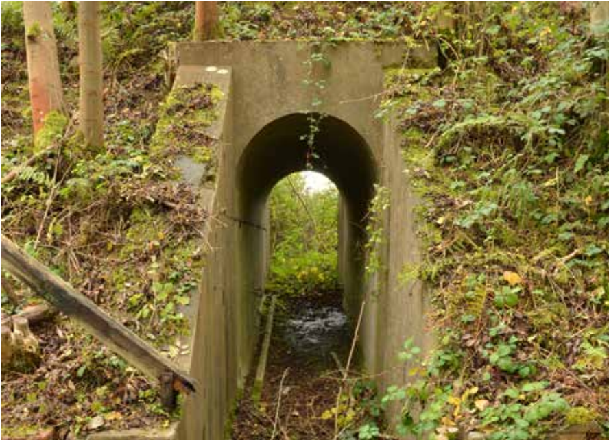
Escape tunnel from the Nitrating House through a bund © Crown
