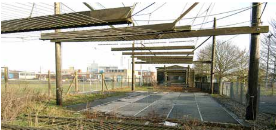
Phased Electromagnetic Simulators shortly before demolition © Crown
