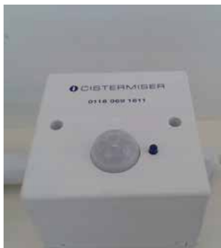
Cistermiser Infrared Control (IRC) unit. © Crown
