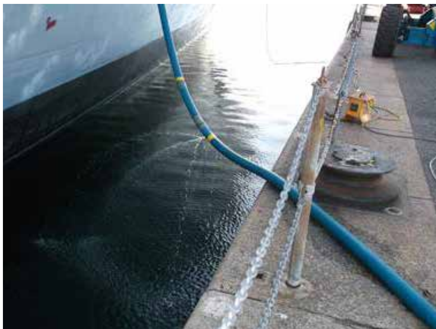
A ship to shore pipe leaking fresh water into the dock area © Paul Morgan
