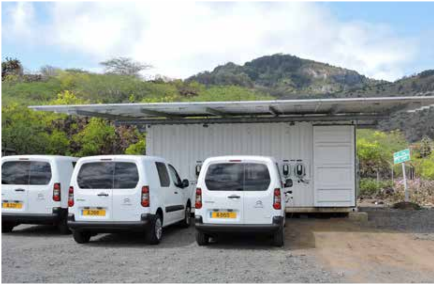
Ascension Island solar powered electric vehicles © Interserve Support Services
