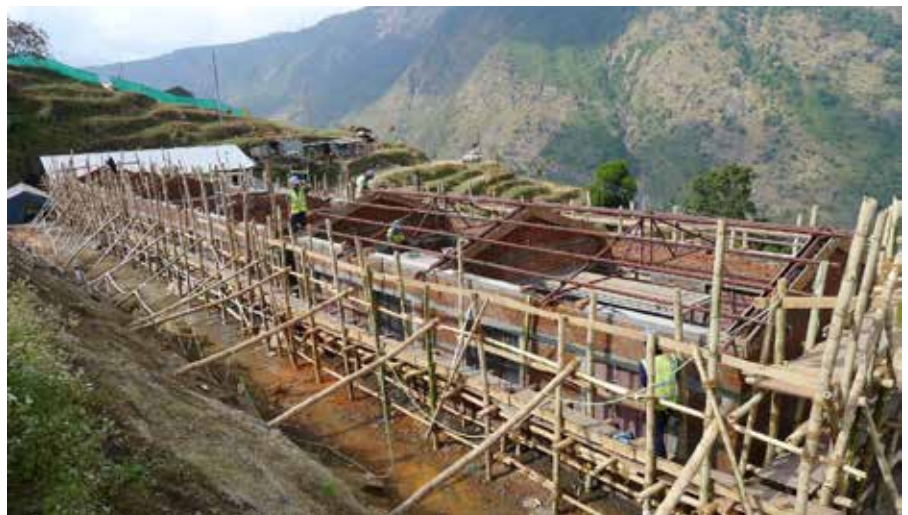
Bamboo scaffolding around the school © Crown
