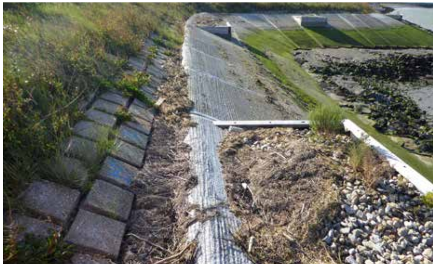
Eco-terraces designed by CH2M as part of the environmental mitigation strategy © QinetiQ
