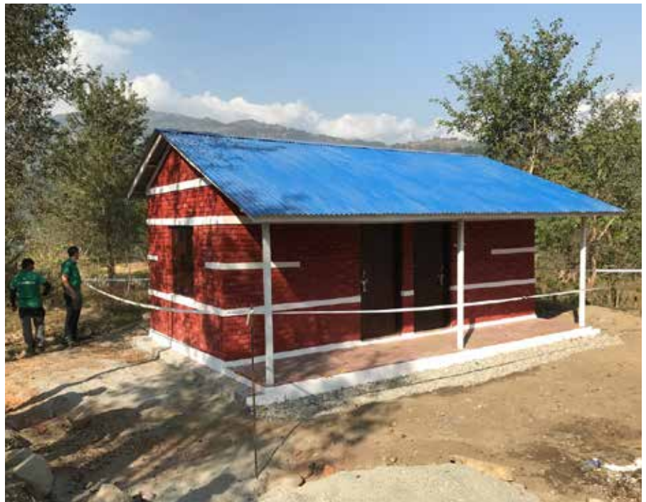
A completed pensioner's home © Crown
