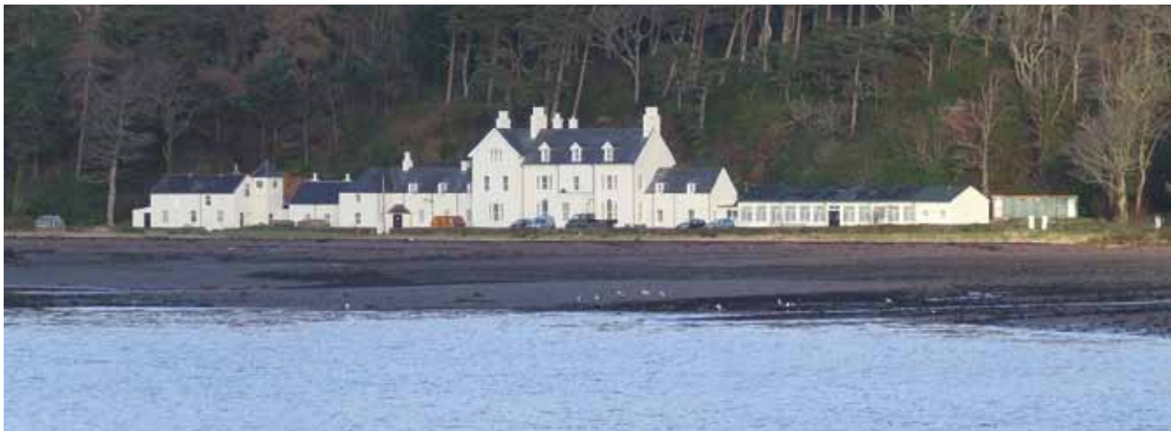
Final tidy up after works complete © Stephen Hudson, Turner Estate Solutions Ltd
