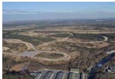
BTA AFV Driver Training Area - tank manoeuvre area and metaled driving circuit © Crown
