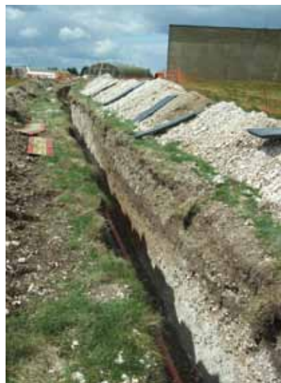
Open trench showing ditch in 2010 © Mike Stone
