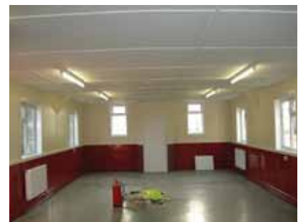
Completed refurbished timber hut © Landmarc
