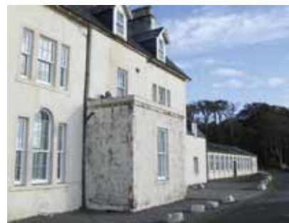
Prior to works © Stephen Hudson, TES
