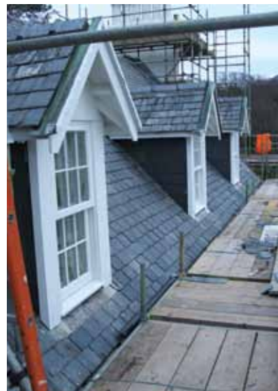
Finishing being applied © Stephen Hudson, TES
