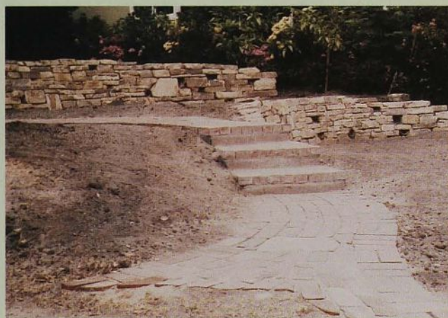
The author designed stone walls and a curving walkway to provide structure to the barren yard of this garden in Carmel.
