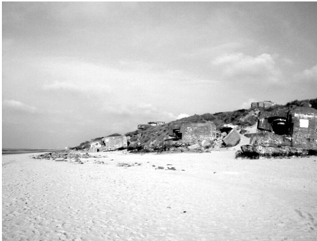
Fig. 2. German bunkers on the upper beach, Leffrinckoucke.
