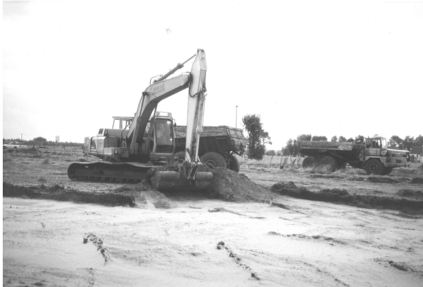
Fig. 3. 1999: The excavating of a fertilised area in D'Heye at Bredene to restore '2190 humid dune slacks' and '2150 EU-Atlantic decalcified fixed dunes ( Callunoa-Ulicetea )'.
