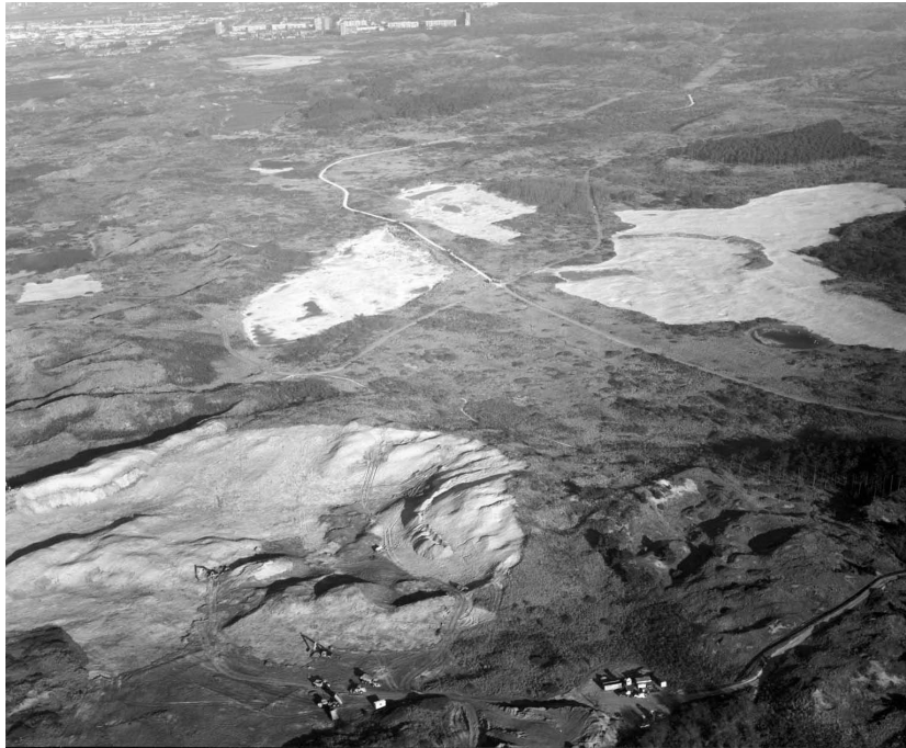
Fig. 5. Work being done in the 'Bride of Harlem'.
