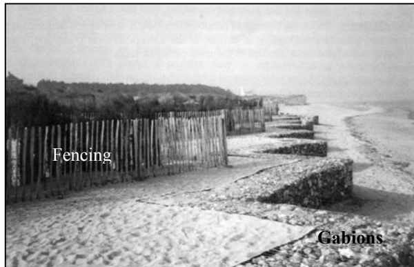
Fig. 3. 'Protected' dunes – gabions and fencing, New Jersey shore, USA.
