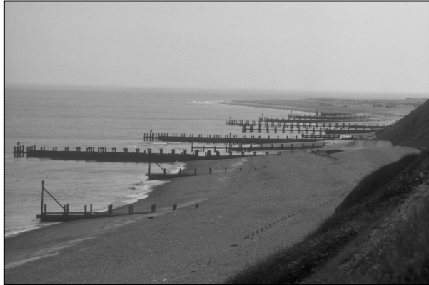
Fig. 8. Kessingland beach looking south from OS Grid. Ref. NR 536870, June 1984. Notice in the foreground how the groyne is showing signs of being covered by shingle.
