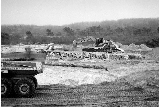
Fig. 6b. The demolition of the Swimming Pool-complex.
