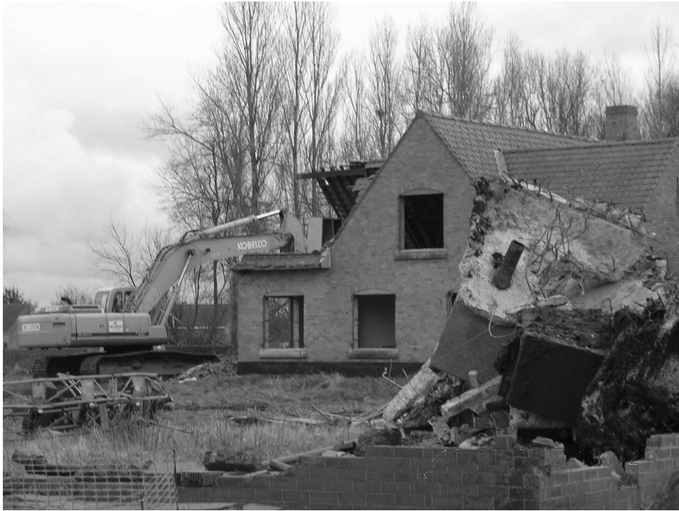
Fig. 7b. The demolition of the derelict water treatment plant at Groenendijk.
