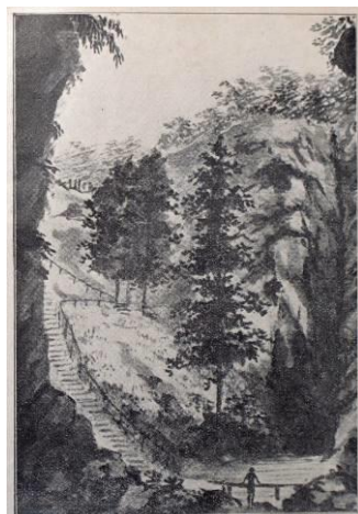
Fig. 2: Technical design of the staircase in the Hranice Abyss by J. H. A. Gallaš in 1816 (Skutil, 1934).
