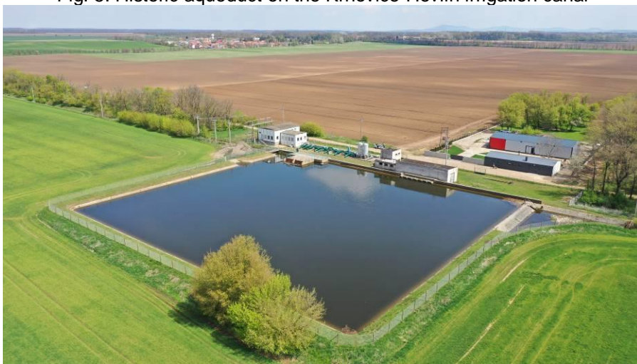
Fig. 6: Water reservoir and water filling station Závlahy Dyjákovice, spol. s r.o.
