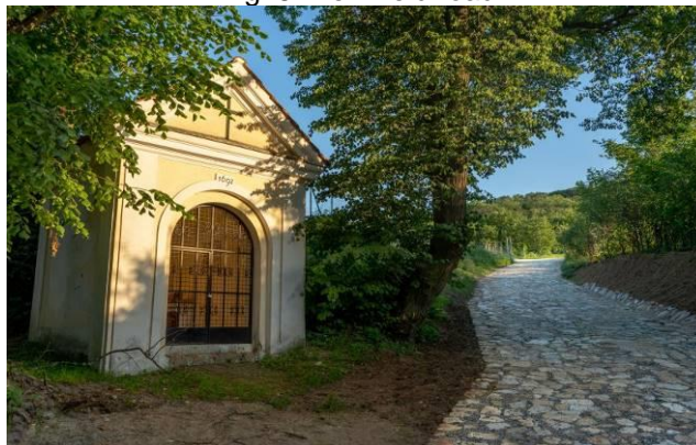
Fig. 9: Detail of the road
