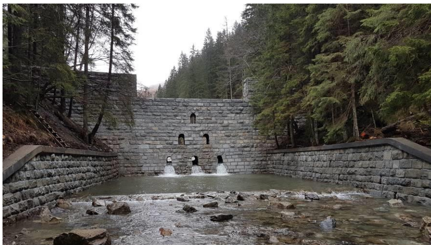
Fig. 2: Stone dam in Račková torrent after reconstruction in 2018–2019
