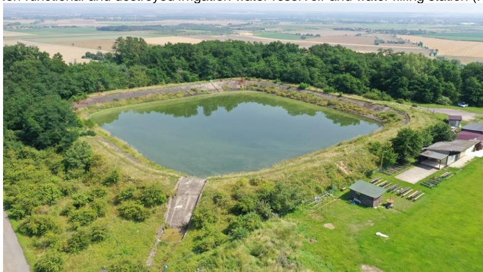
Fig. 10: Non-functional irrigation water reservoir (Brandýs nad Labem)
