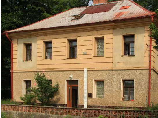
Fig. 2: Hadík ferry – ferryman's house with historical flood markers
