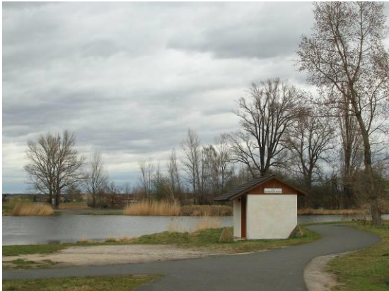
Fig. 4: Záryby – preserved ferryman's house
