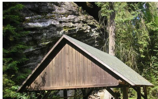
Fig. 5: Asphalt shingle roofing
