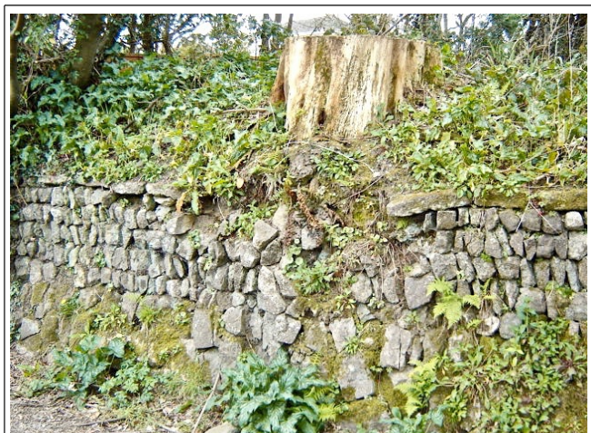
This old tree has been left until the hedge structure is damaged and the stump, cut down too short, has died.
