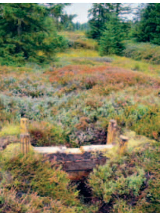
/ A dam across a drainage ditch increasing the water table as part of a restoration scheme in the Vraký peatland in the northwestern part of the country near the border with Germany. Photo: Jana Jiskrová
