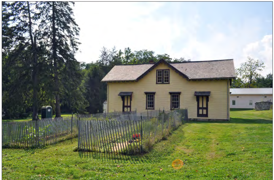
Figure 3.40. Garden Maintenance Building. Fenced cold frame foundations are visible in the foreground and the new Collections Storage Building is visible to the right. View looking west, 2013 (OCLP).
