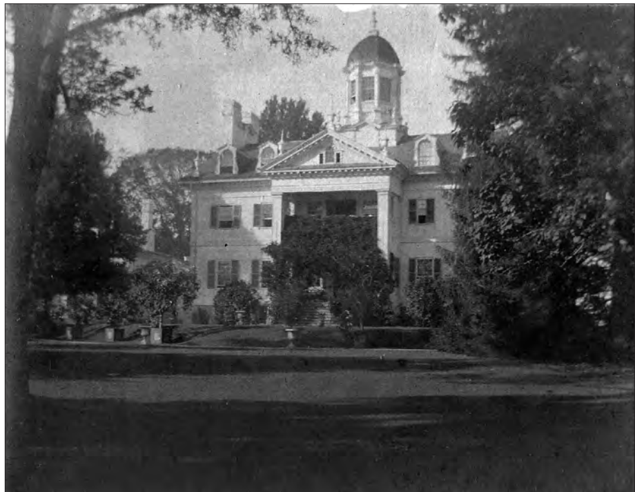
Figure 1.37. Gelatin print of the south facade of the Hampton Mansion from the Great Terrace. View looking north, c. 1900 (HAMP 18583).
