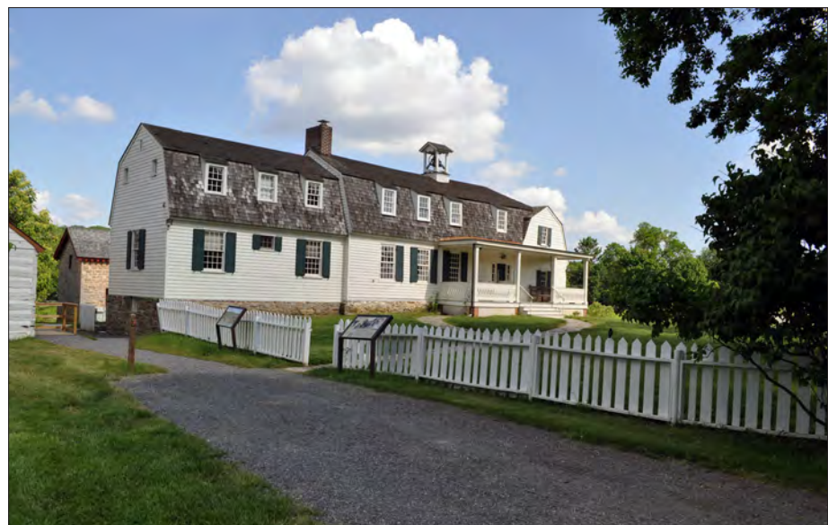
Figure 3.88. West facade of the Farm House from Farm Road. View looking southeast, 2012 (OCLP).
