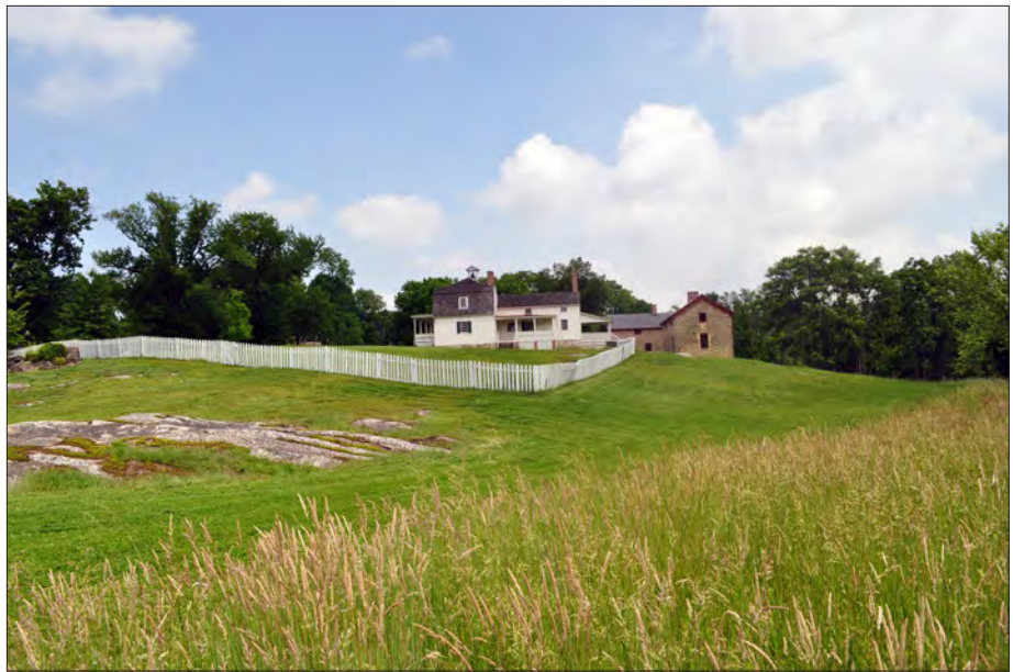
Figure 0.4. The Farm House Cluster from the Dairy stream. View looking north, 2012 (OCLP).
