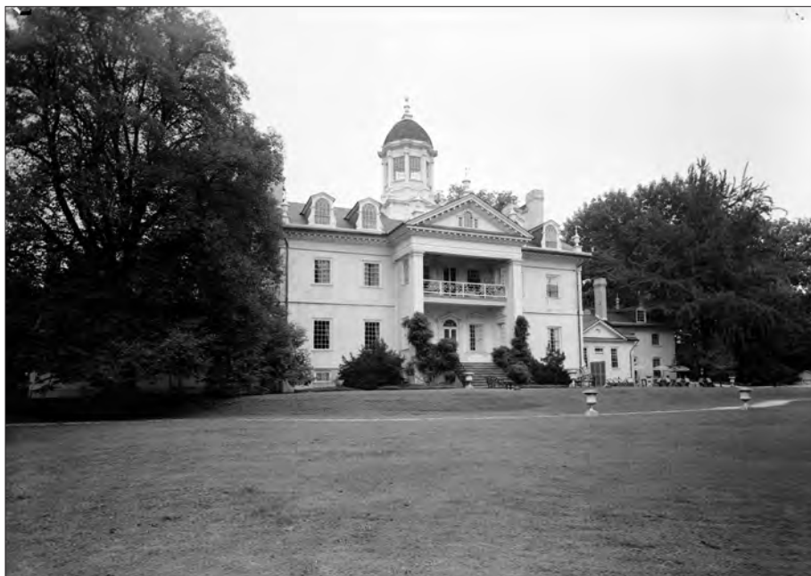
Figure 1.96. Hampton Mansion, with wisteria climbing the south portico. Note the Tea Room concession tables and umbrellas to the right of the Mansion. View looking northeast, 1959 (HABS MD-226-A, Lanny Miyamoto).
