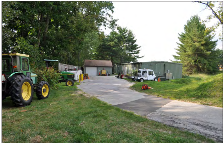
Figure 3.50. The Park Maintenance Building with white garage door (on the left) from the maintenance parking area. View looking northwest, 2013 (OCLP).
