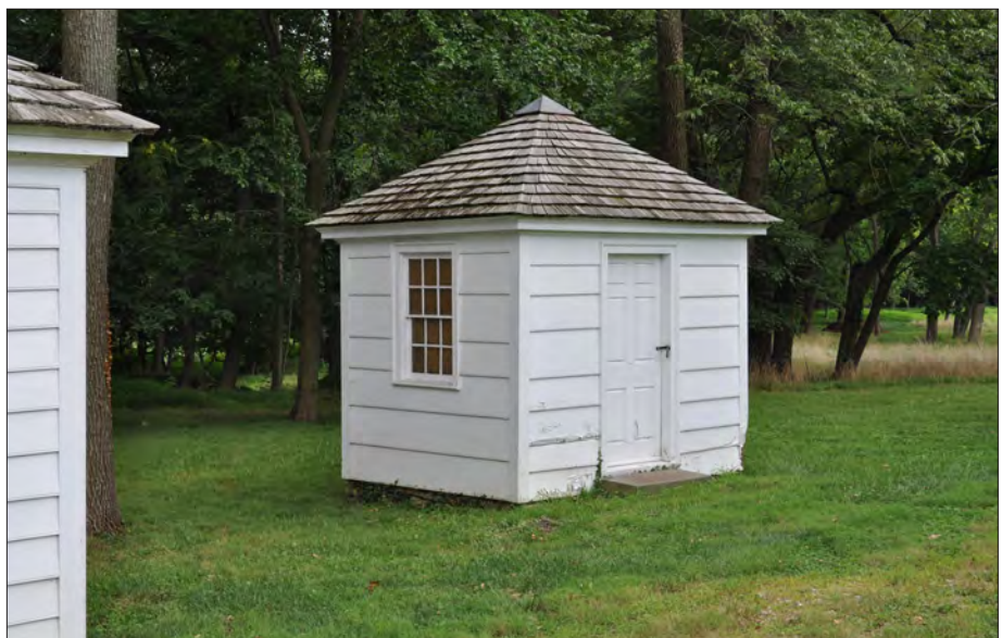
Figure 3.52. Privy #1. View looking southeast, 2013 (OCLP).
