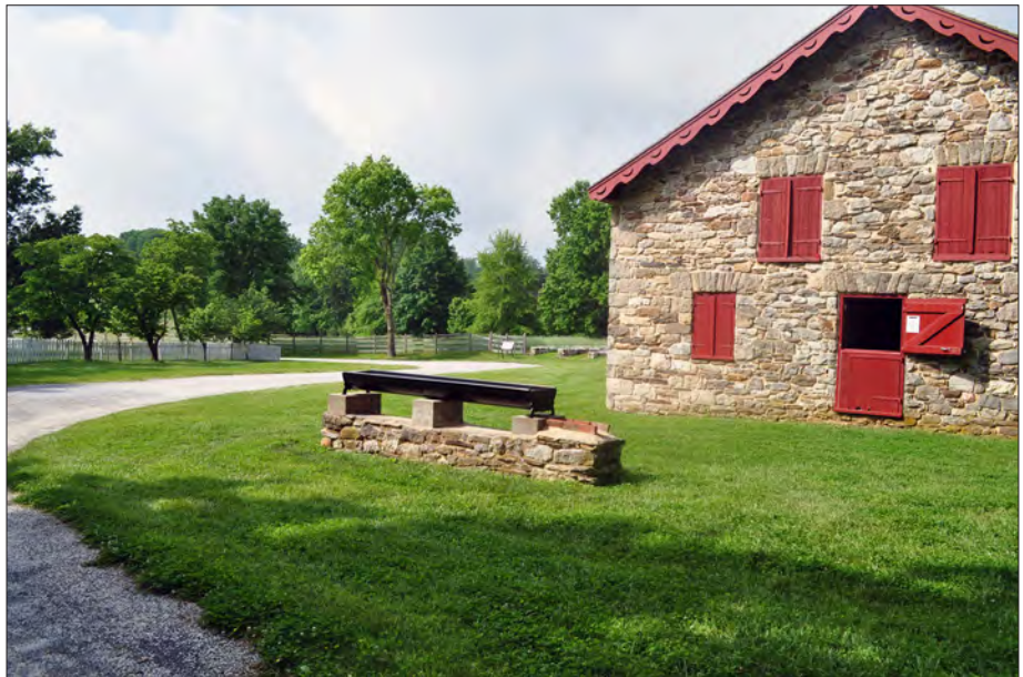
Figure 3.102. Mule Barn trough, with the Mule Barn visible to the right. View looking southwest, 2012 (OCLP).
