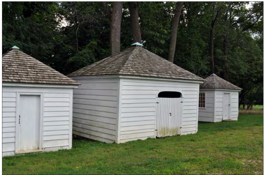
Figure 3.49. Paint House at center. The Smoke House is on the left and Privy #1 is on the right. View looking southeast, 2013 (OCLP).
