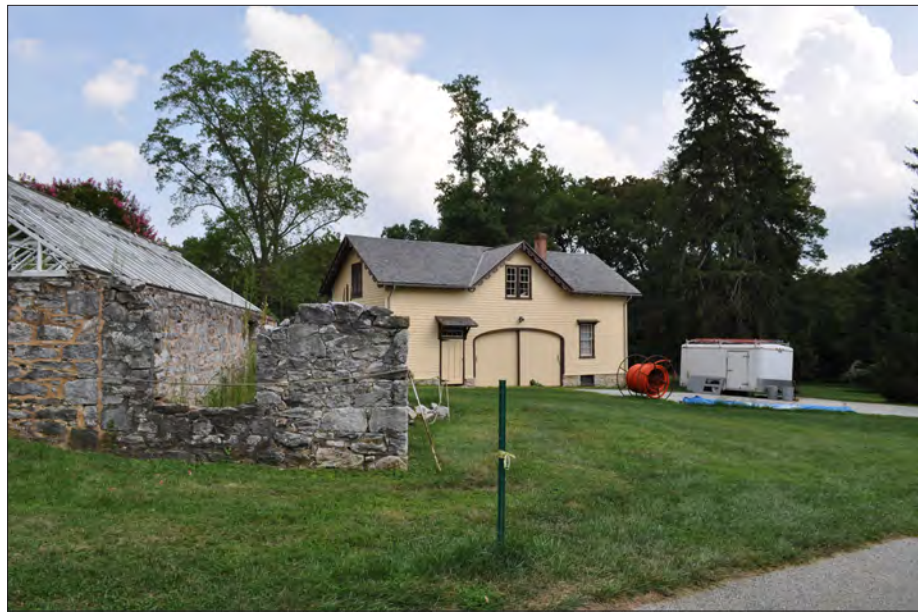
Figure 3.5. Garden Maintenance Area. View looking southeast, 2013 (OCLP).
