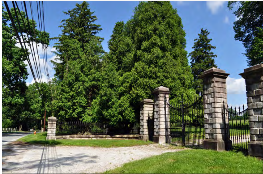
Figure 3.66. Mansion gates from Hampton Lane. View looking east, 2012 (OCLP).
