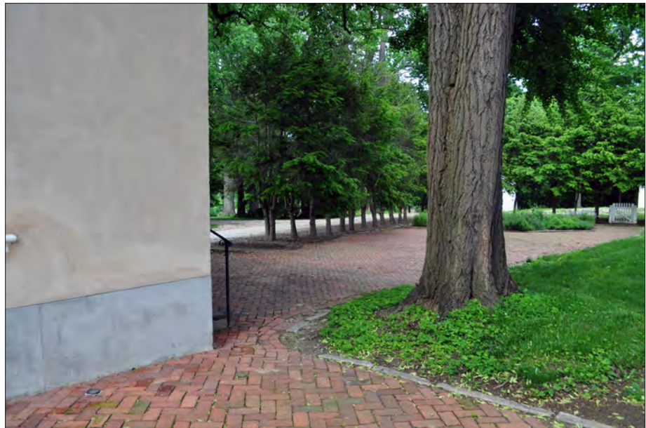
Figure 3.23. East Terrace from the Brick Terrace at the southwest corner of the Mansion. View looking northeast, 2012 (OCLP).
