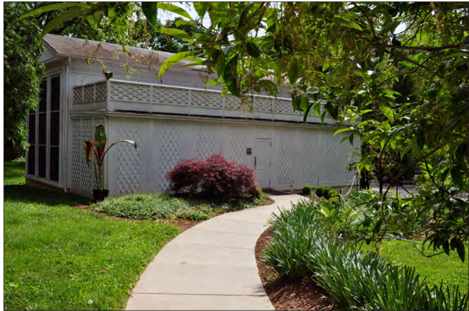
Figure 3.30. Concrete walk leading to the Orangerie from the historic entrance drive. View looking southwest, 2012 (OCLP).
