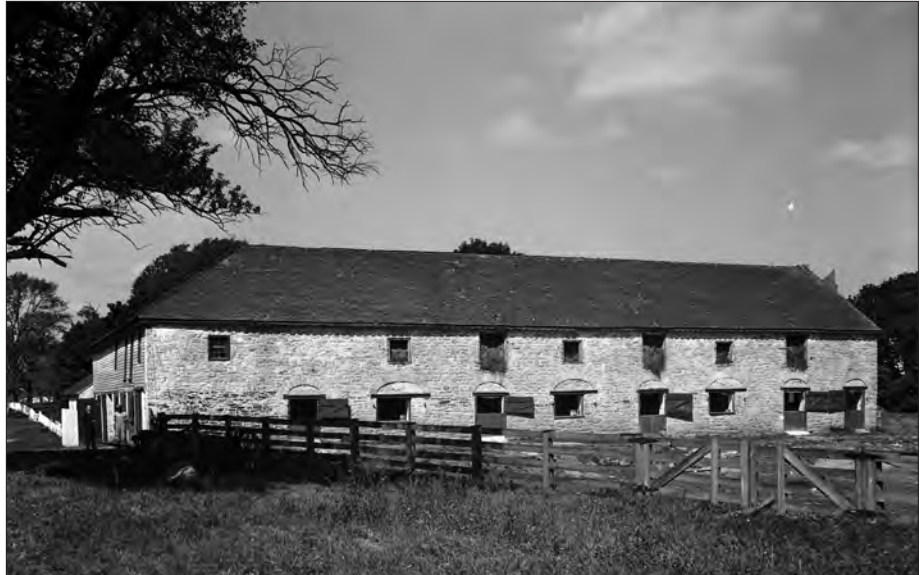
Figure 1.50. Cow Barn, with the Long House Granary visible beyond at left. View looking northwest, 1936 (HABS MD-22-6H, E.H. Pickering).
