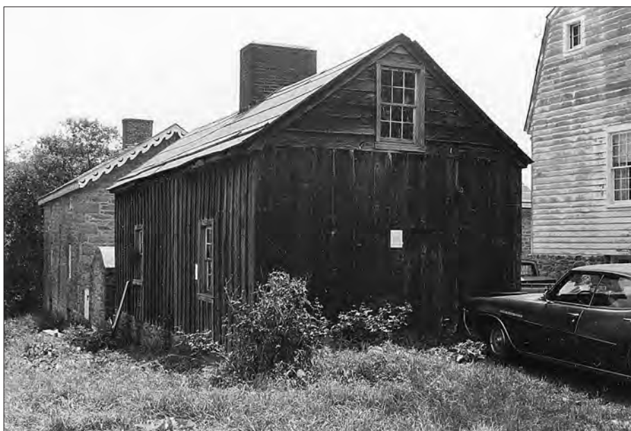
Figure 1.92. Log Farm Structure with the Farm House to the right and Salve Quarters #2 beyond. View looking south, c. 1970 (HAMP15482).
