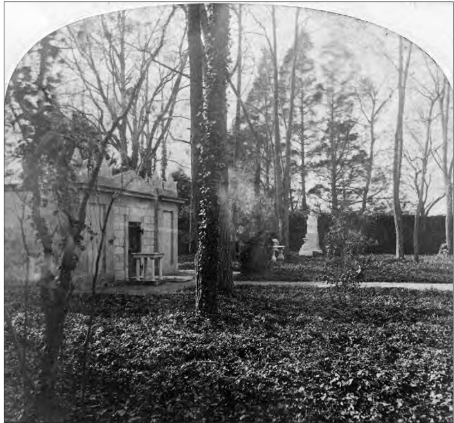
Figure 1.33. Stereograph of the Ridgely Family Cemetery showing the Ridgely Family Vault at left. View looking southwest, 1872 (HAMP 20236).
