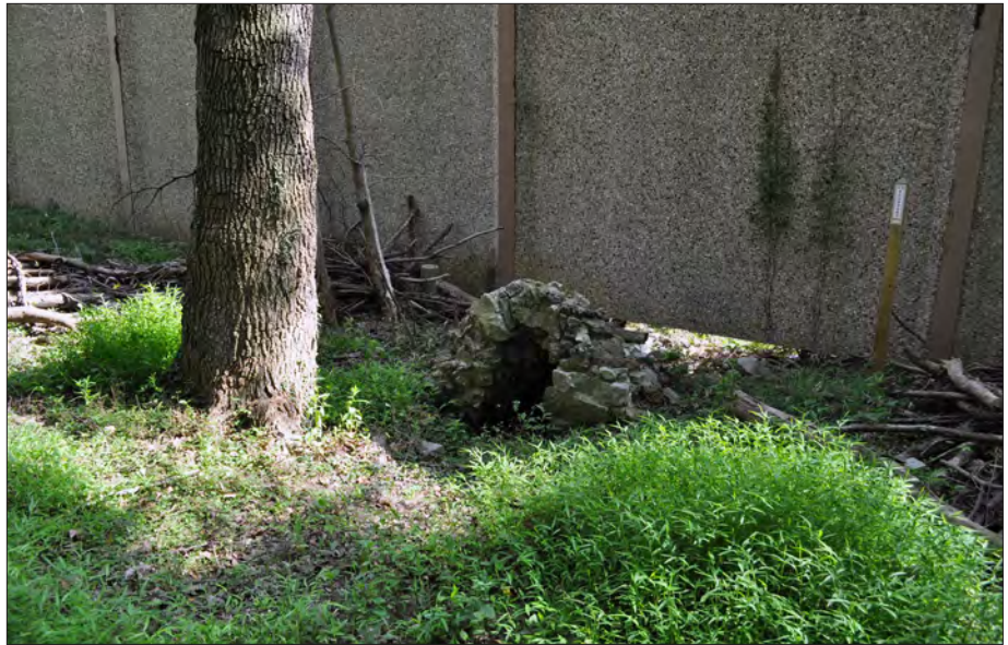
Figure 3.57. South Spring ruin. View looking south, 2013 (OCLP).
