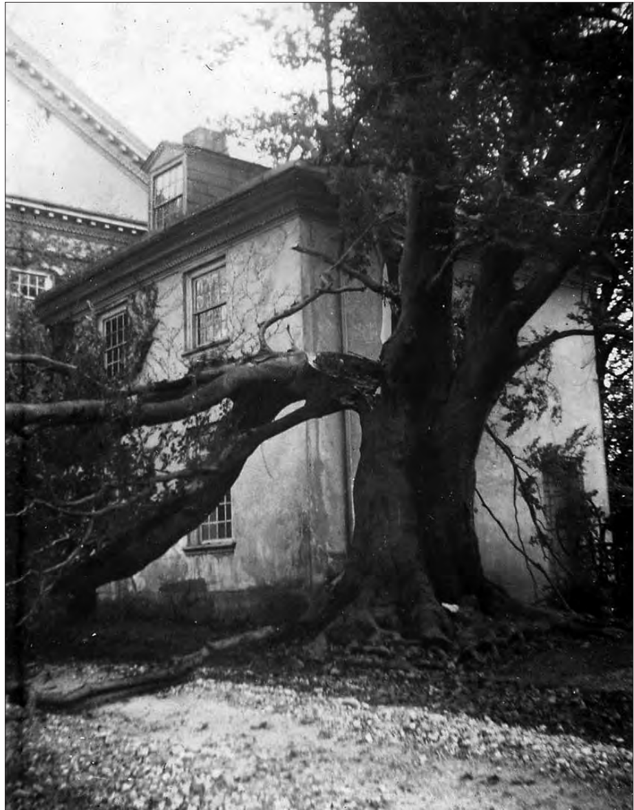
Figure 1.86. West wing of the Hampton Mansion showing a storm damaged purple-leaved European beech tree. View looking southeast, 1940 (HAMP 18146).
