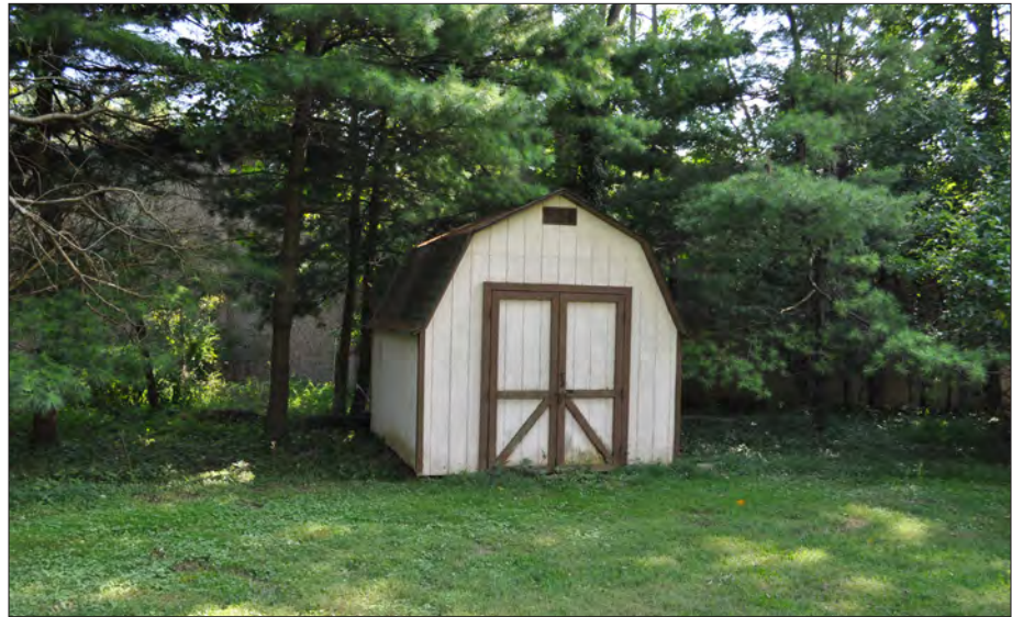
Figure 3.37. Caretaker's Shed. View looking south, 2013 (OCLP).
