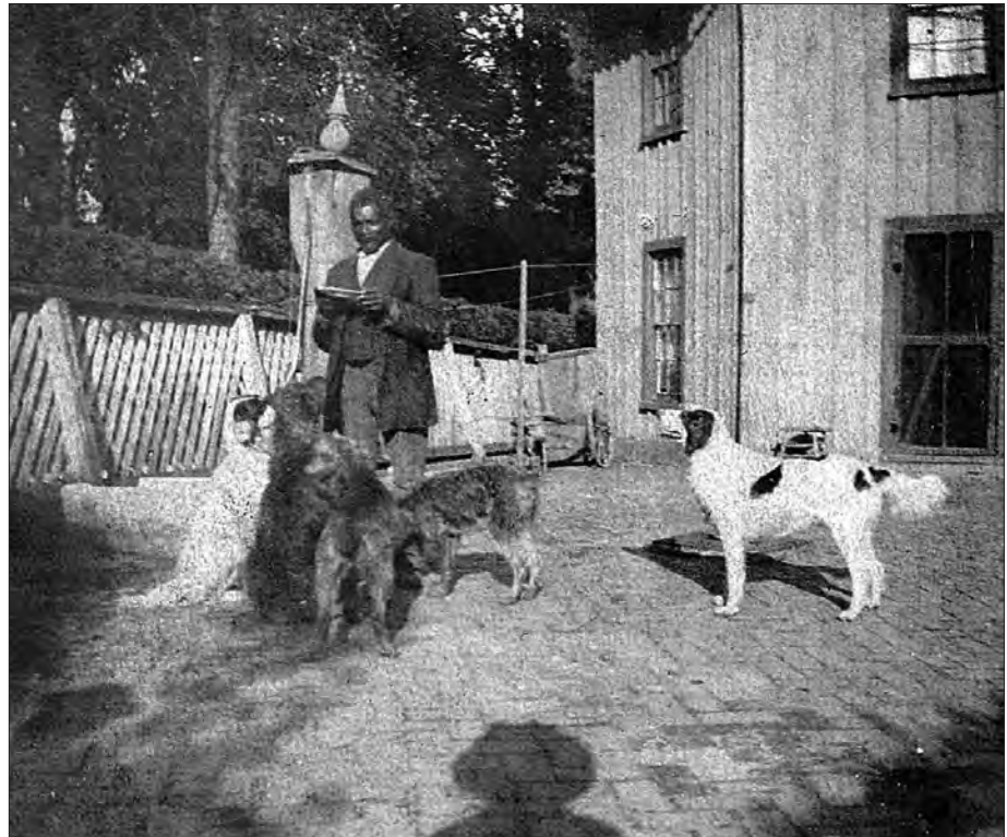
Figure 1.67. The East Terrace showing the lattice fence that bordered the north side of the terrace. View looking northeast, c. 1913 (HAMP 6365).
