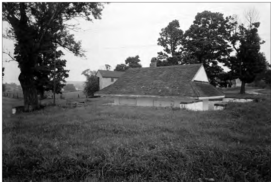
Figure 1.91. The Dairy from Farm Road. View looking east, 1959 (HABS MD-226-F, Lanny Miyamoto).
