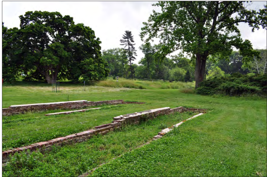
Figure 3.63. Cold frame foundations to the east of the Caretaker's Cottage. View looking east, 2012 (OCLP).
