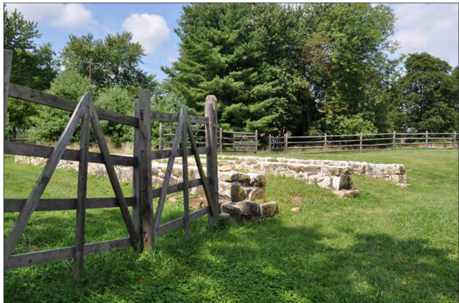
Figure 3.86. Corn Crib foundation, with the West Farm Field fence visible to the left. View looking northwest, 2013 (OCLP).
