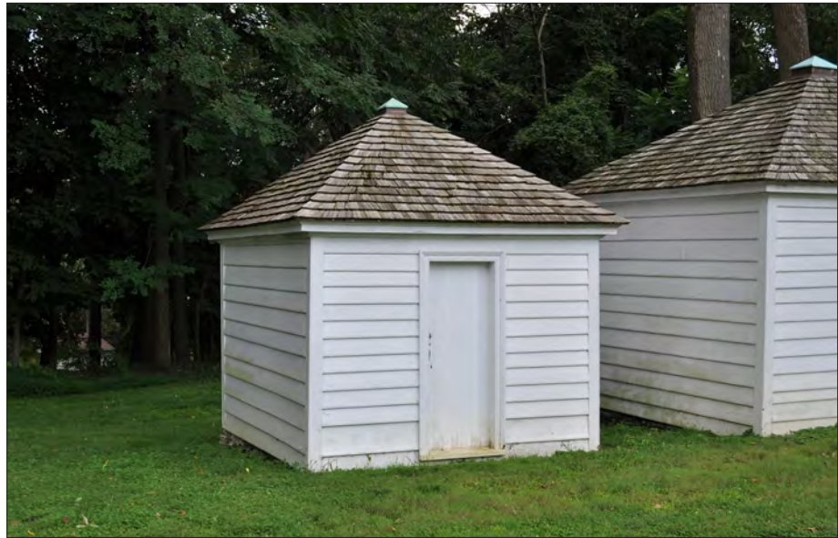
Figure 3.56. Smoke House (left), adjacent to the Paint House (right). View looking southeast, 2013 (OCLP).
