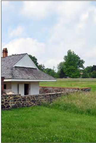
Figure 0.1. The Hampton Dairy. View looking west, 2012 (OCLP).
