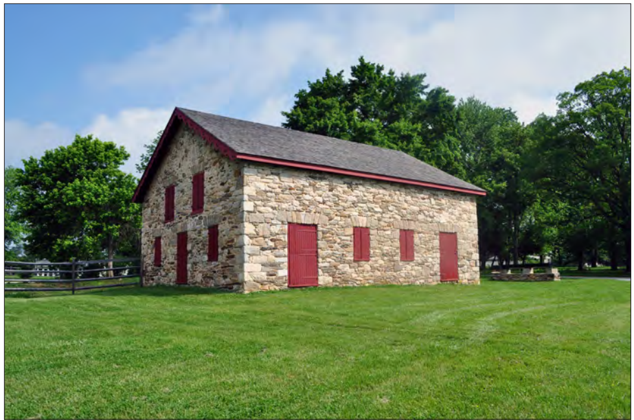
Figure 3.91. Mule Barn from Farm Road. View looking northwest, 2012 (OCLP).
