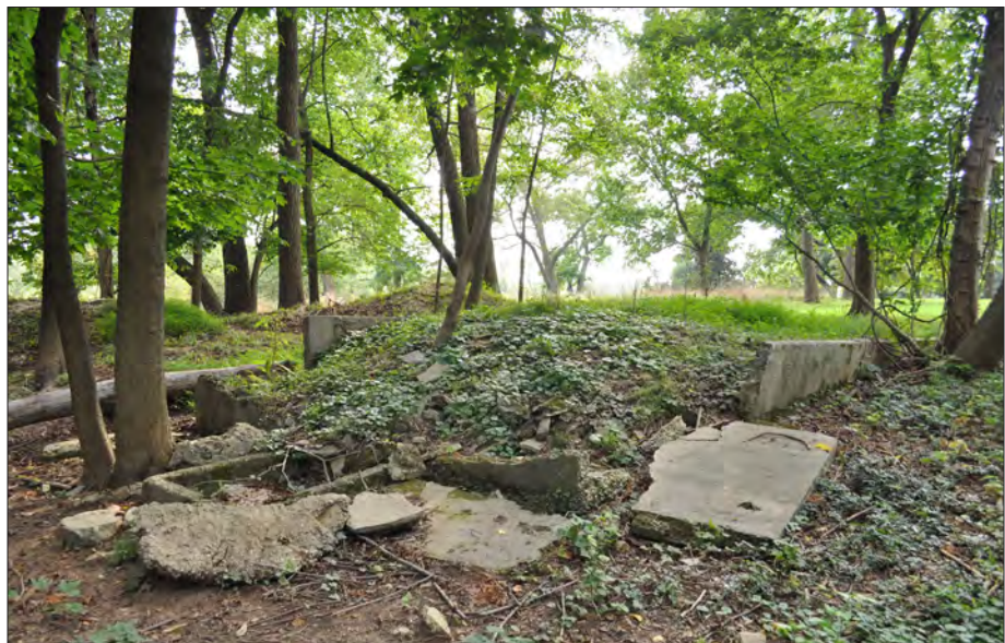
Figure 3.51. Site of the Pole Barn foundation. View looking west, 2013 (OCLP).
