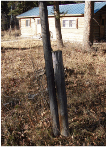
Early electric pole: base supported by extra post. Source: Utah State University.
