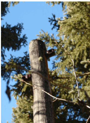
Early electric pole: the top, with ceramic insulator. Source: Utah State University.
