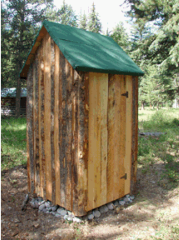
Rebuilt mock outhouse, Aug. 1, 2009. Source: Utah State University.
