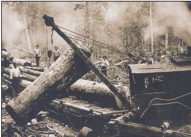
Figure 2.1.1.1. A steam-powered loader uses tongs to place logs onto a railroad flat car in the Smokies in the early 1900s.
