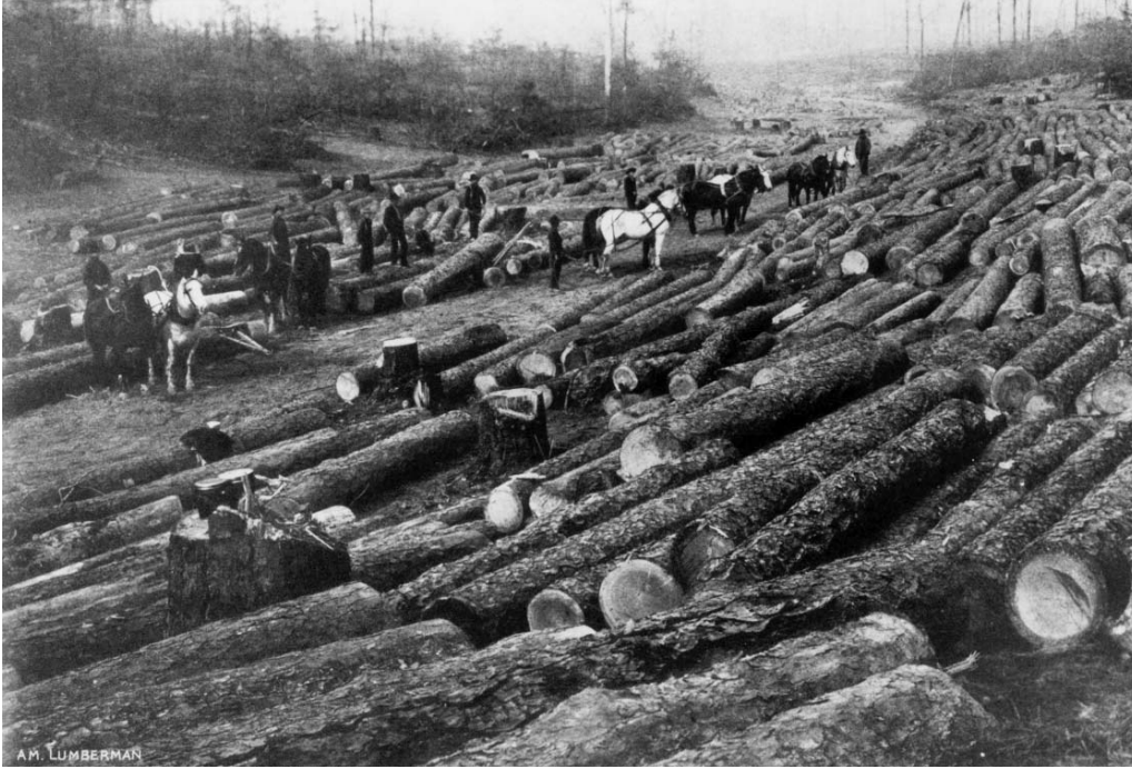
FIGURE 14. Clearing right-of-way through virgin longleaf forest in Mississippi for the Natchez, Columbia and Mobile Railroad in 1907. All timber was soon cut within several miles of railroads and more distant lands were sold to logging companies. Photo, American Lumberman 1907.
