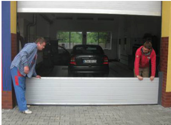
Fig. 2 Mobile protection on the garage door. Source Roman Konieczny
