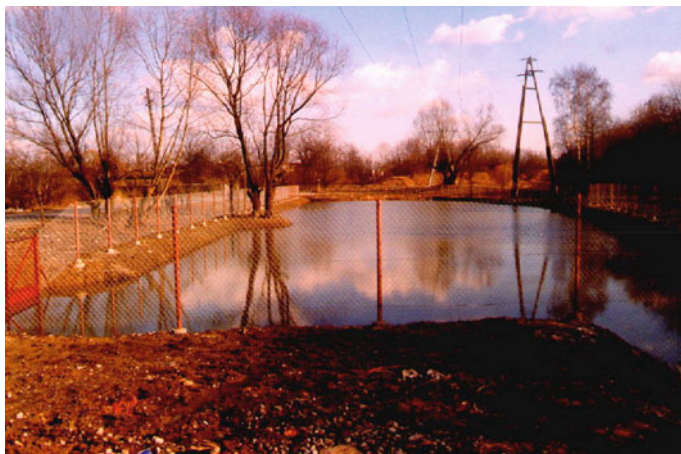
Fig. 6 Wet stormwater pond constructed to collect surface runoff from paved surfaces in a housing estate in Kraków
