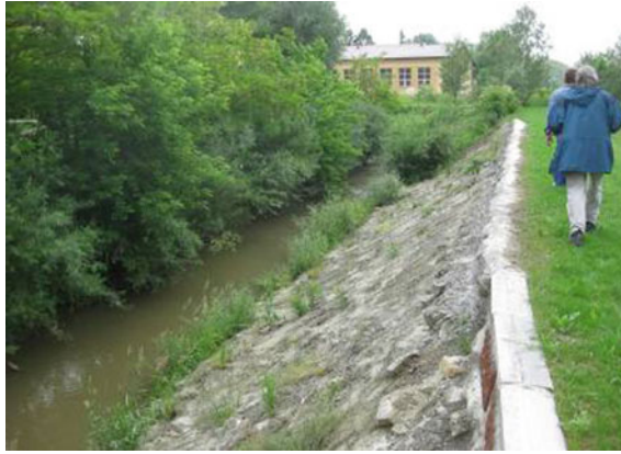
Fig. 1 Reinforced stream bank. Source Małgorzata Siudak
