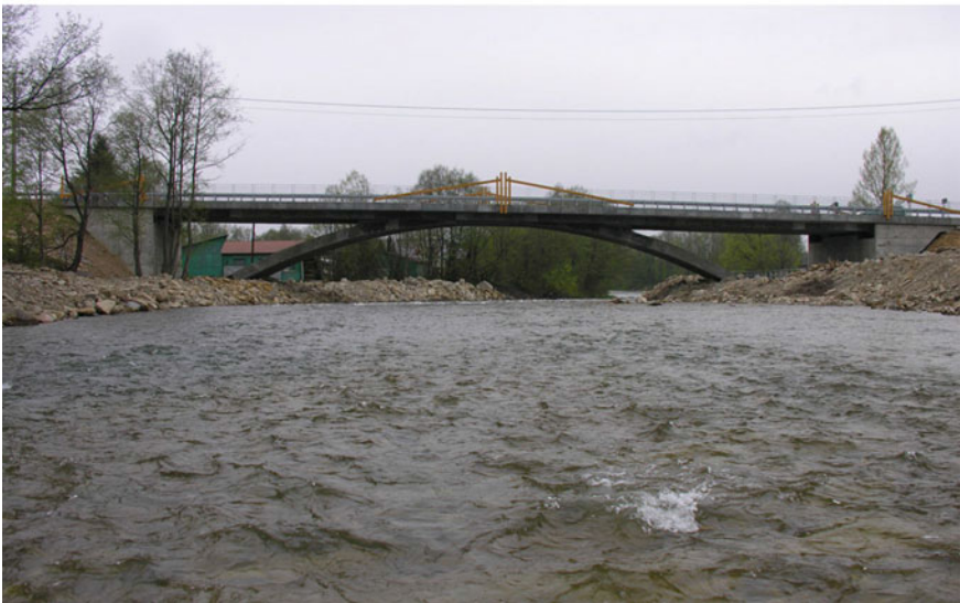
Fig. 9 a Bridge on the Czarny Dunajec River at Chochółów before 2005, with its piers based on the channel bed. During the flood of 2001 wood jams were deposited on the upstream side of the piers, reducing cross-sectional area of the flow. b The bridge at Chochółów rebuilt in 2005. The arch supporting the new bridge is based outside the river channel, which excludes a possibility of channel obstruction by deposited woody debris. After Wyżga and Radecki-Pawlik (2011)
